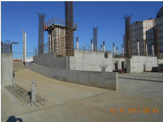
Ramp and walls level 1 at Transportation Bldg.
