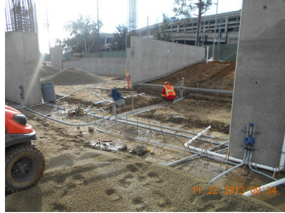
Installation of UG conduits and water pipes at Garage Bldg.
