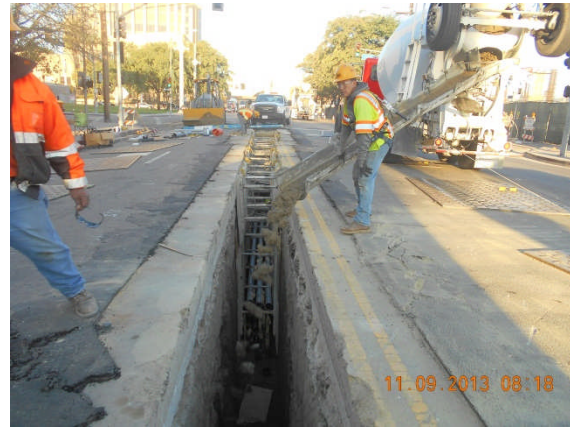
Slurry placement in UG trench at Cesar Chavez Avenue.
