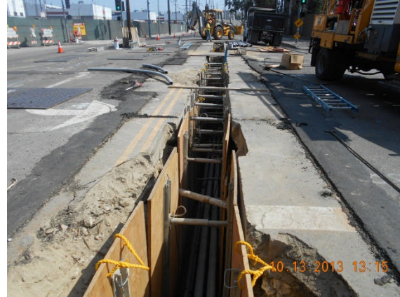
Underground electrical conduit installation at Cesar Chavez.
