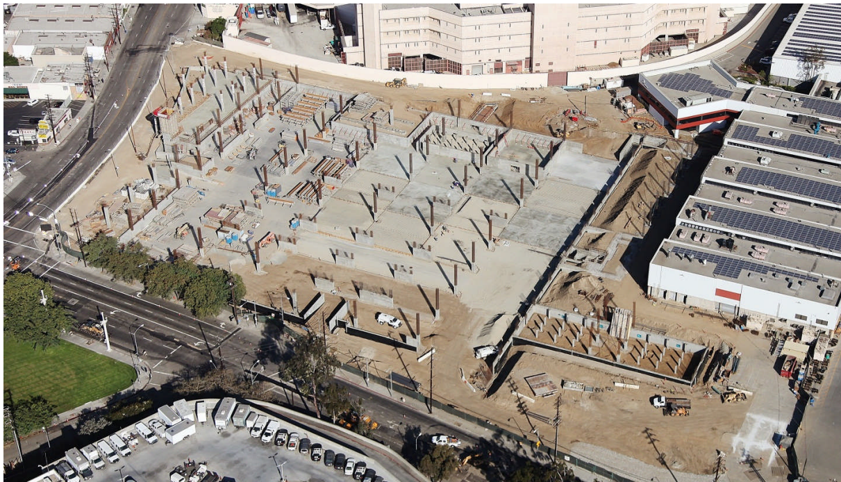
Transportation Building, Parking Garage and Maintenance Building in construction; at the bottom side Cesar Chavez Avenue and at the left side Vignes Street – December 2013.
