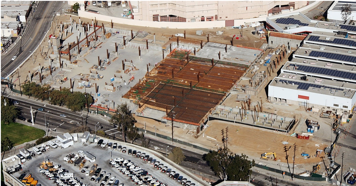
Transportation Building, Parking Garage and Maintenance Building in construction; at the bottom side Cesar Chavez Avenue and at the left side Vignes Street – October 2013.
