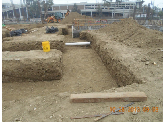
Footing excavation and rebar placement at Areas 8, 9, 10.
