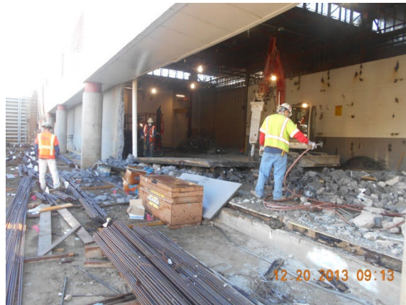
Demolition of CMU wall at old Radiator Shop.
