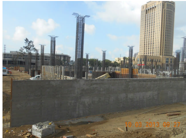
Reservoir tank concrete walls at Parking Garage.
