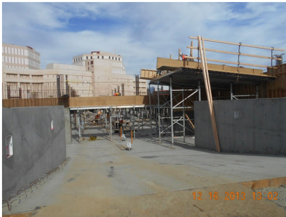
Formwork setting for elevated ramp 1 st level Parking Garage.
