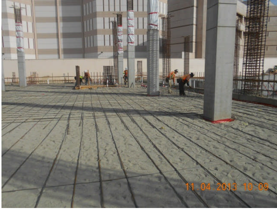
Rebar placement for slab on grade at Transportation Bldg.
