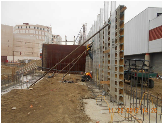
Formwork setting of south east wall at level 1 Area 9.
