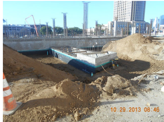
Fan room underground tunnel concrete walls in progress.
