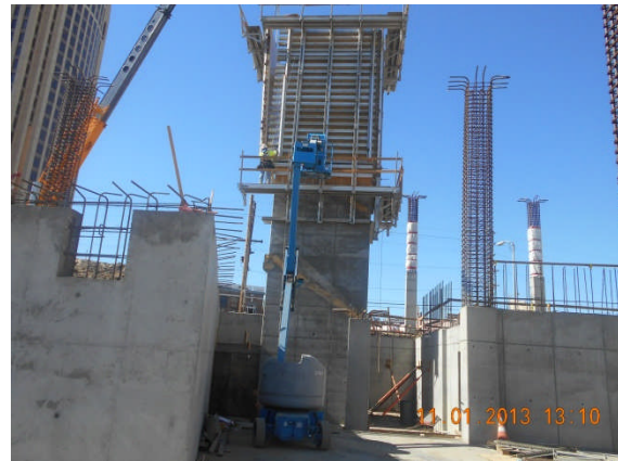
Setting of wall formwork for elevator No. 1 shaft at Area 1.
