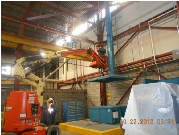
Exhaust duct placement at new Radiator Shop.
