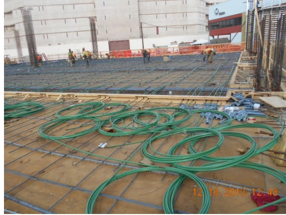
Steel rebar and tendon placement on 1 st level deck at Area 7.
