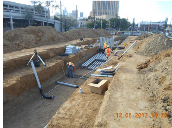
Installation of UG elec. conduits for main duct bank Area 8.
