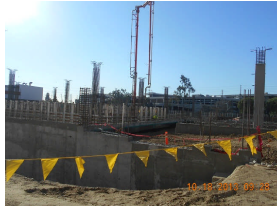
Concrete wall placement in progress at Area 7.
