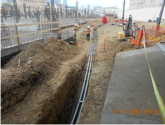
Installation of UG electrical conduits at Metro Driveway.
