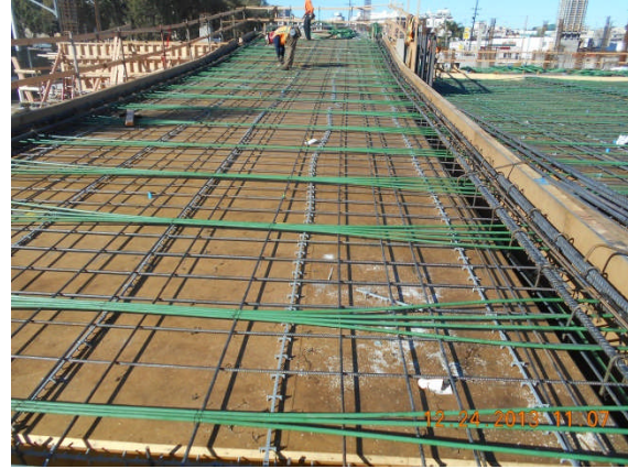
Tendons placement at elevated ramp of Garage Building.
