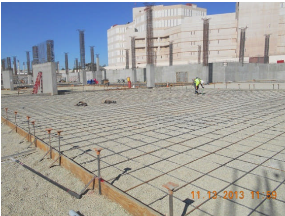
Rebar placement on lower level at Areas 6 and 7.
