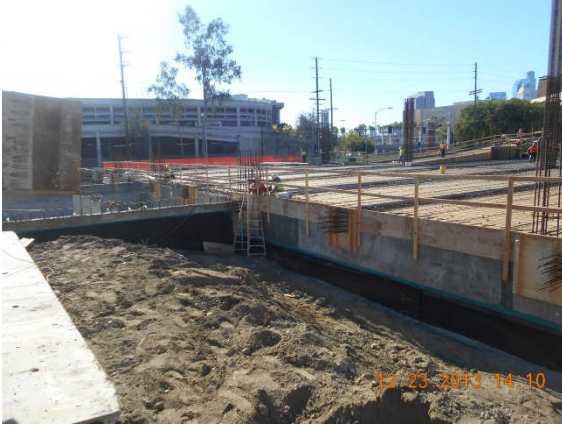
Placement of steel rebar for beams 1 st level deck Area 5.
