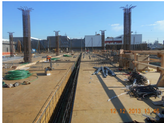
Steel rebar and tendons placement 1 st level deck at Area 7.
