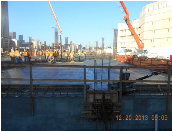
First pour of 1 st level deck at Area 7 Parking Garage.
