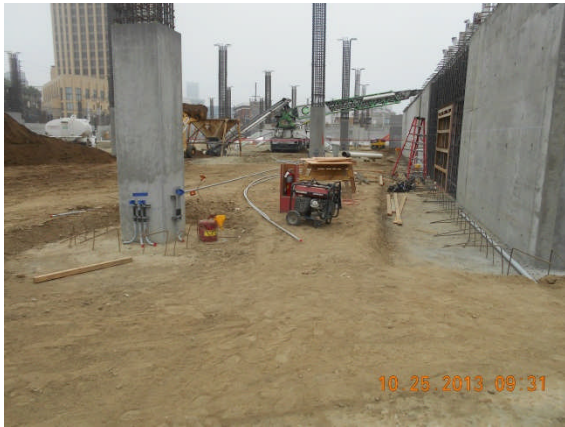
Wall concrete placement at Brake Room in progress.
