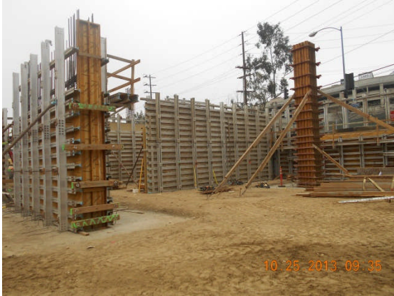
Lower level form walls at Area 5 in progress.
