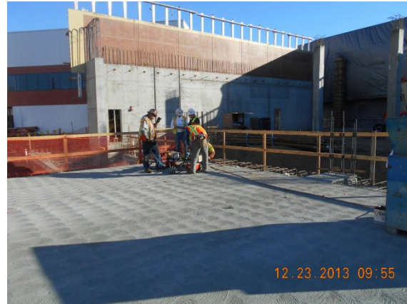
Pulling of tendons in concrete slab at 1 st level deck Area 7.
