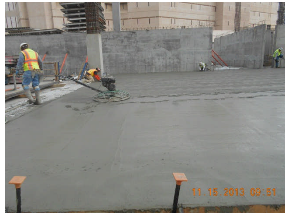
Concrete slab finish on lower level at Area 7.
