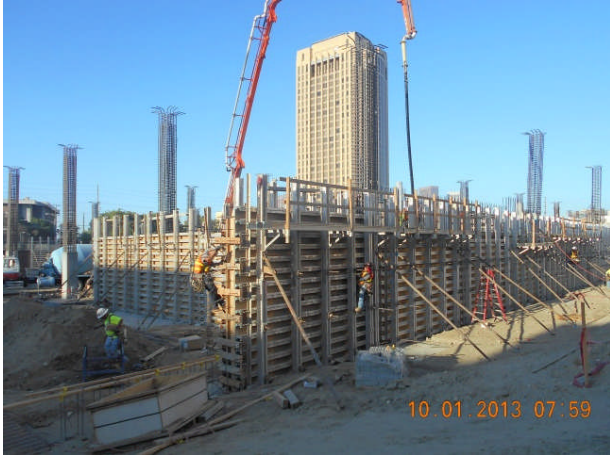
Walls concrete placement for reservoir tank on Building B.
