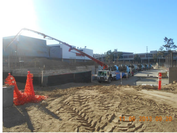
Concrete pour for foundations and footings at Areas 8-9.
