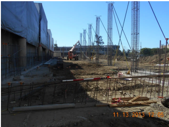
Columns erection at Areas 8 and 9.
