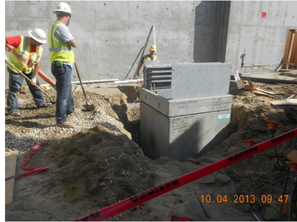
Oil water vault installation at Parking Garage.
