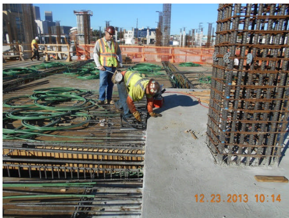
Monitoring and testing of tendon pulling on 1 st level deck.
