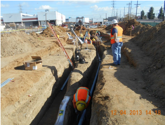
Excavation for underground electrical conduits at Area 8.
