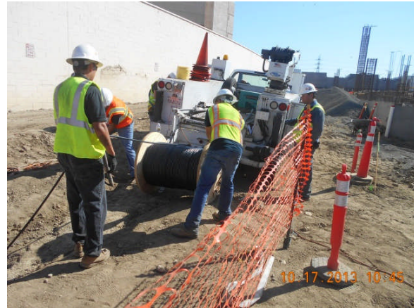
Fiber optic installation in progress on Metro Driveway.
