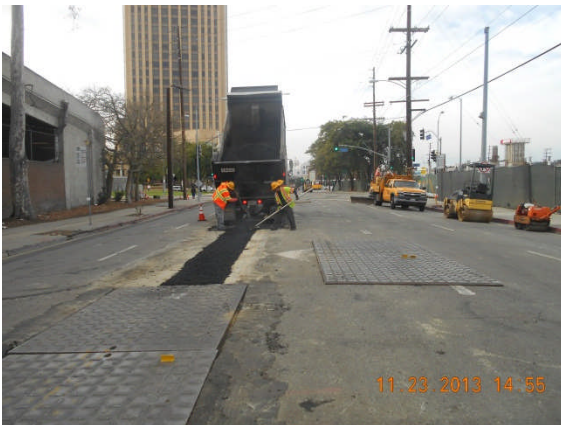
AC patch of UG trench at Cesar Chavez.
