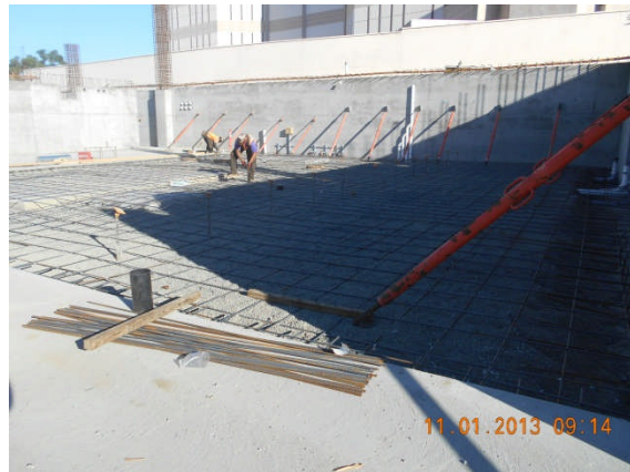
Rebar placement for slab on grade at Area 7 lower level.
