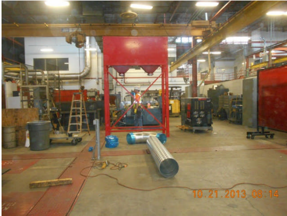
Duct work installation at Plasma Room in progress.
