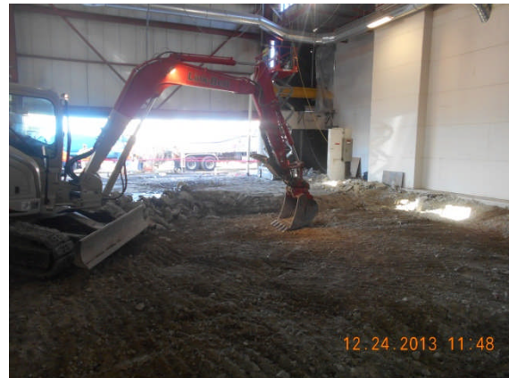
Demolition of existing concrete slab at old Radiator Shop.
