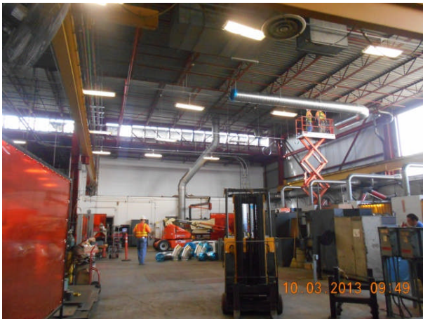
Duct installation for plasma cutter at Weld Shop.
