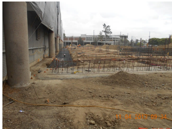
Rebar reinforcement at foundation and footing at Areas 8-9.
