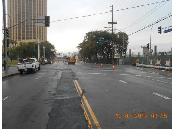
AC patch of UG utilities trench at Cesar Chavez.
