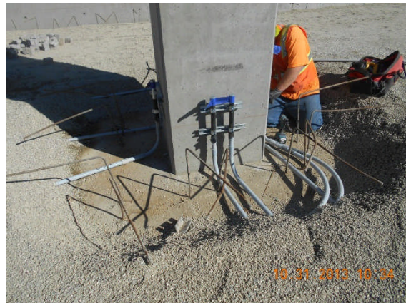
U.G. electrical conduits at column base of Area 5.
