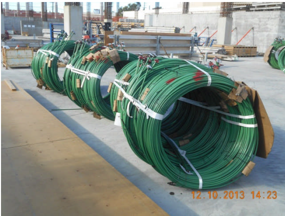
Post tension tendons for deck & beam buildup at 1 st level dk.
