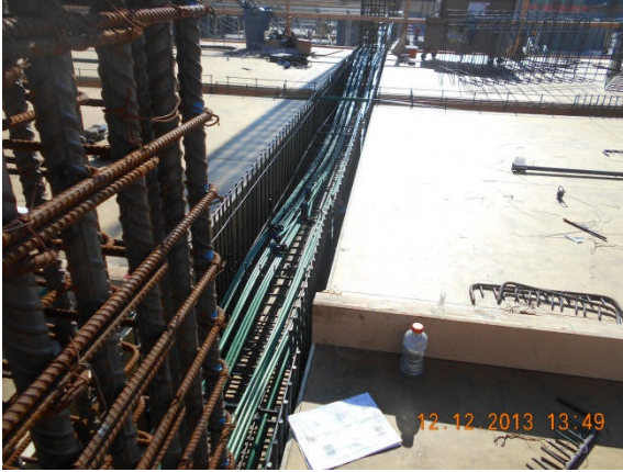
P.T. tendons placement at beams 1 st level deck Area 7.
