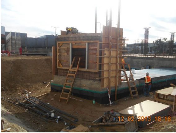
Placement of walls formwork for Exhaust Room.
