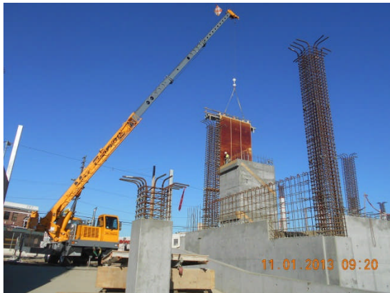
Setting of steel formwork for elevator No. 1 shaft at Area 1.
