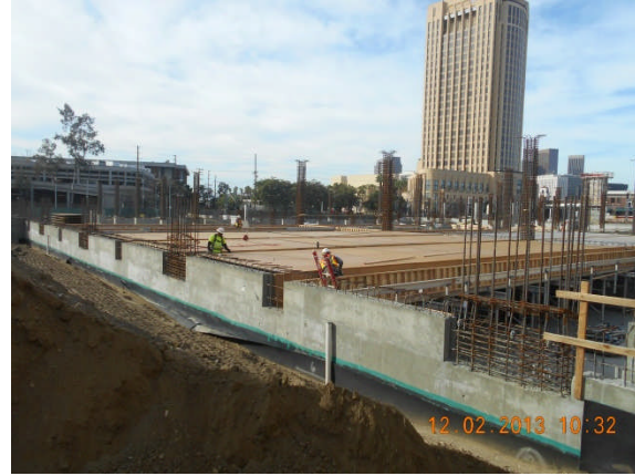
Setting of 1 st level deck panels at Area 7.
