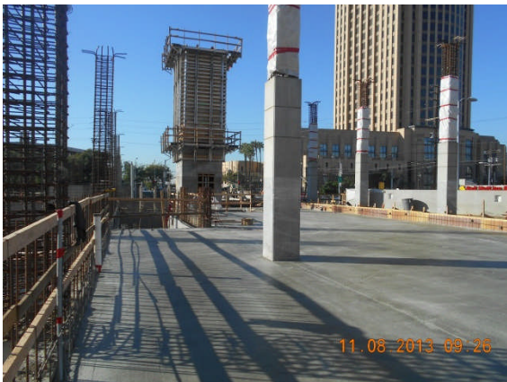
Concrete poured for slab on grade at Transportation Bldg.
