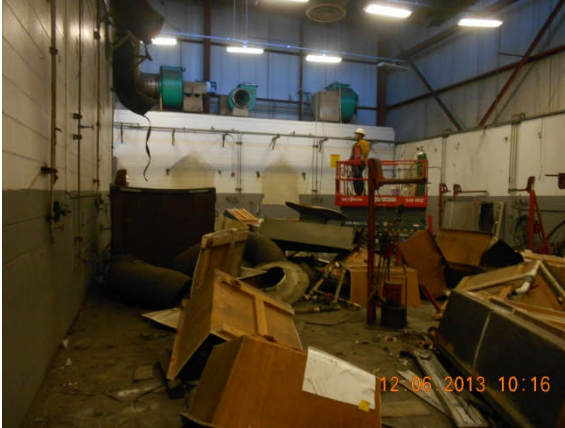
Interior soft demolition of old Radiator Shop.
