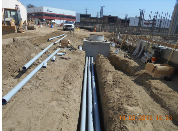
Fiber optic installation on Metro Driveway.
