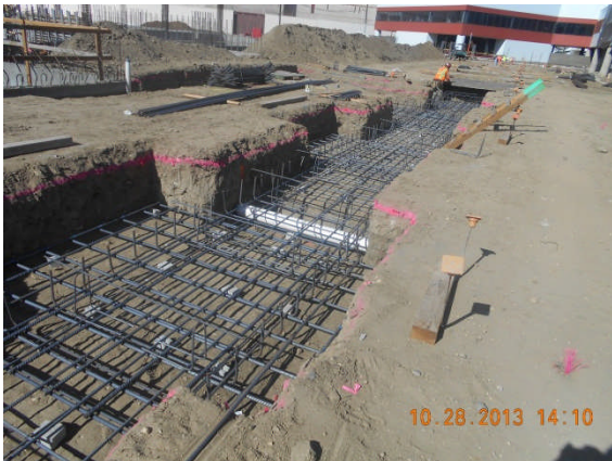
Rebar placement for foundation at Areas 8, 9 and 10.
