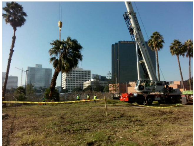
Tree Removal at VA Site
