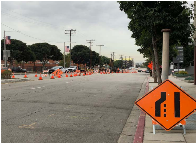
SCG Relocations Temporary Traffic Control Southbound Federal Avenue
