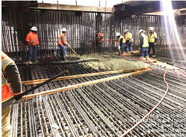
TBM Launch Box Invert Slab in Century City
