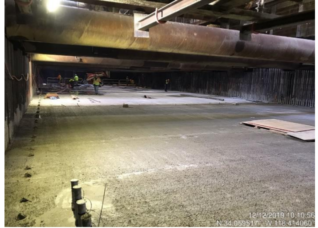
TBM Launch Box Invert Slab in Century City
