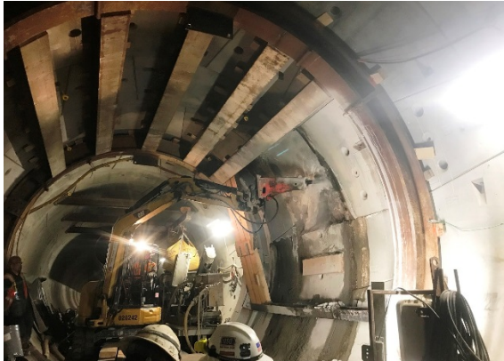
Cross Passage 10 Construction
