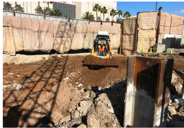
Entrance Appendage Excavation at Wilshire/Fairfax Station
