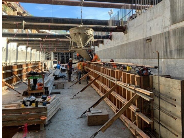
Platform wall placement at the future Little Tokyo/Arts District Station
