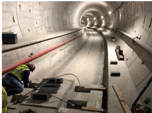
Floating slab installation in the left tunnel
