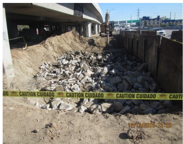
Austin Vault, Excavation
