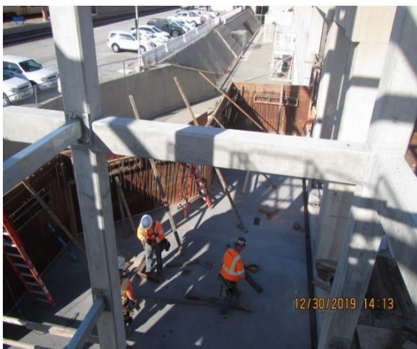
Elevator Platform, Forming the walls.
