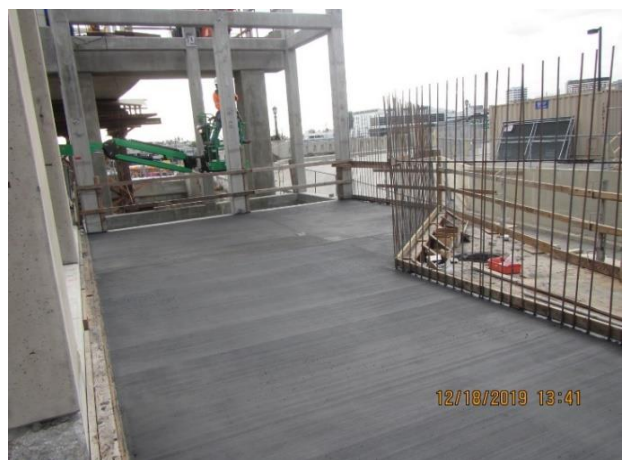
Elevator Platform, Poured
