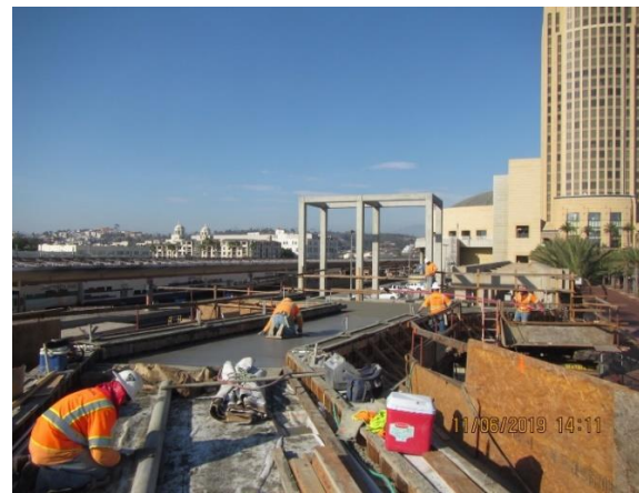
Pedestrian Walkway, poured
