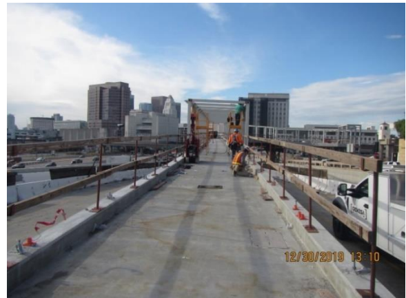
Pedestrian Bridge, Overcrossing & Walkway. Steel frames erection
