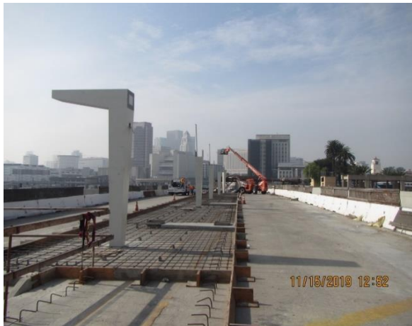
Bus Platform Canopy, Columns installation.
