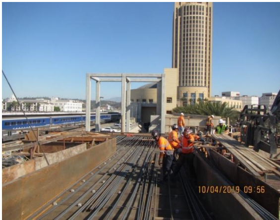
Pedestrian Walkway Rebar
