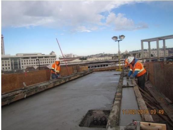
Pedestrian Overcrossing, Poured
