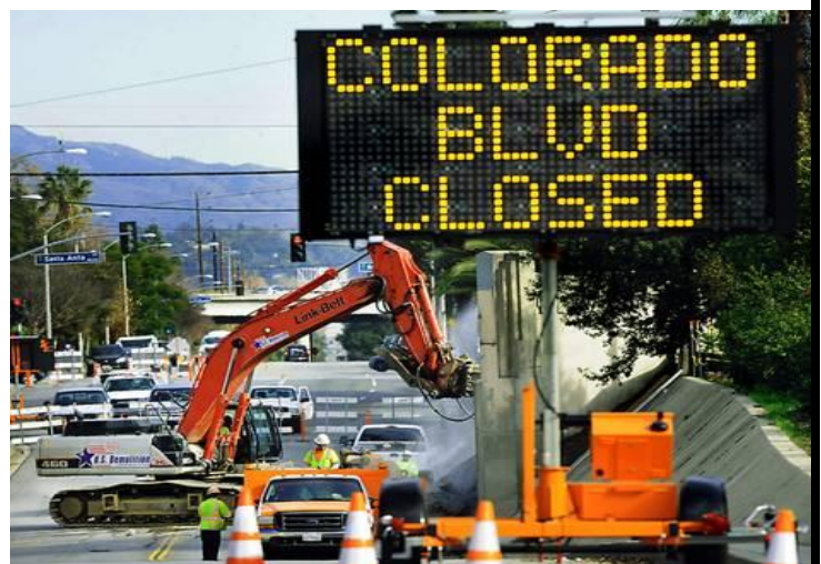
Example of Notices for Colorado Bridge Work
