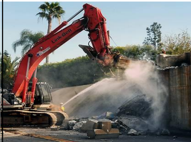
Work at Colorado Bridge
