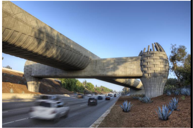
View of finalized bridge
