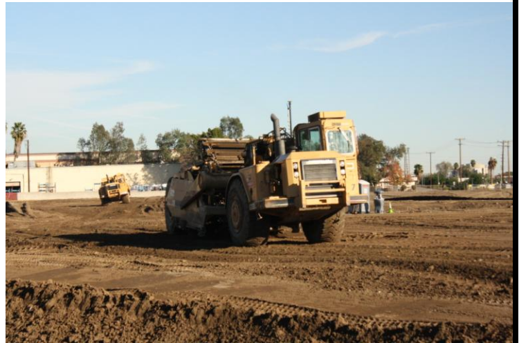
Grading work at Gold Line Operations Campus
