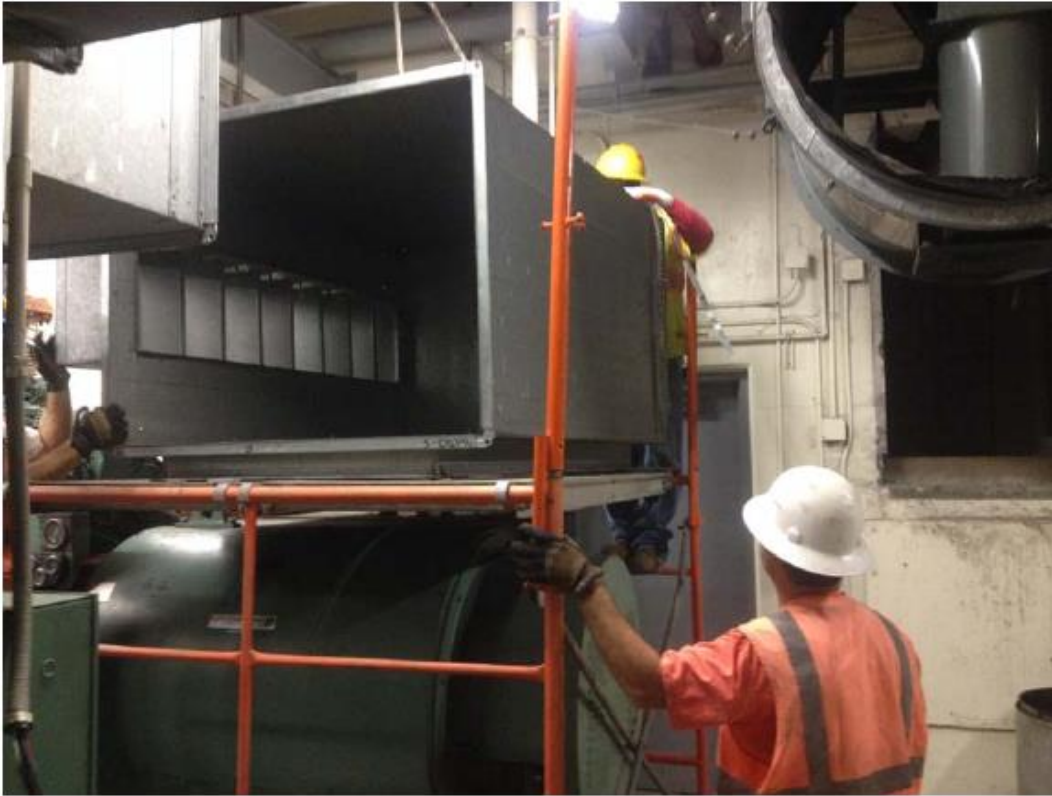
LA Times building basement ducting removal
