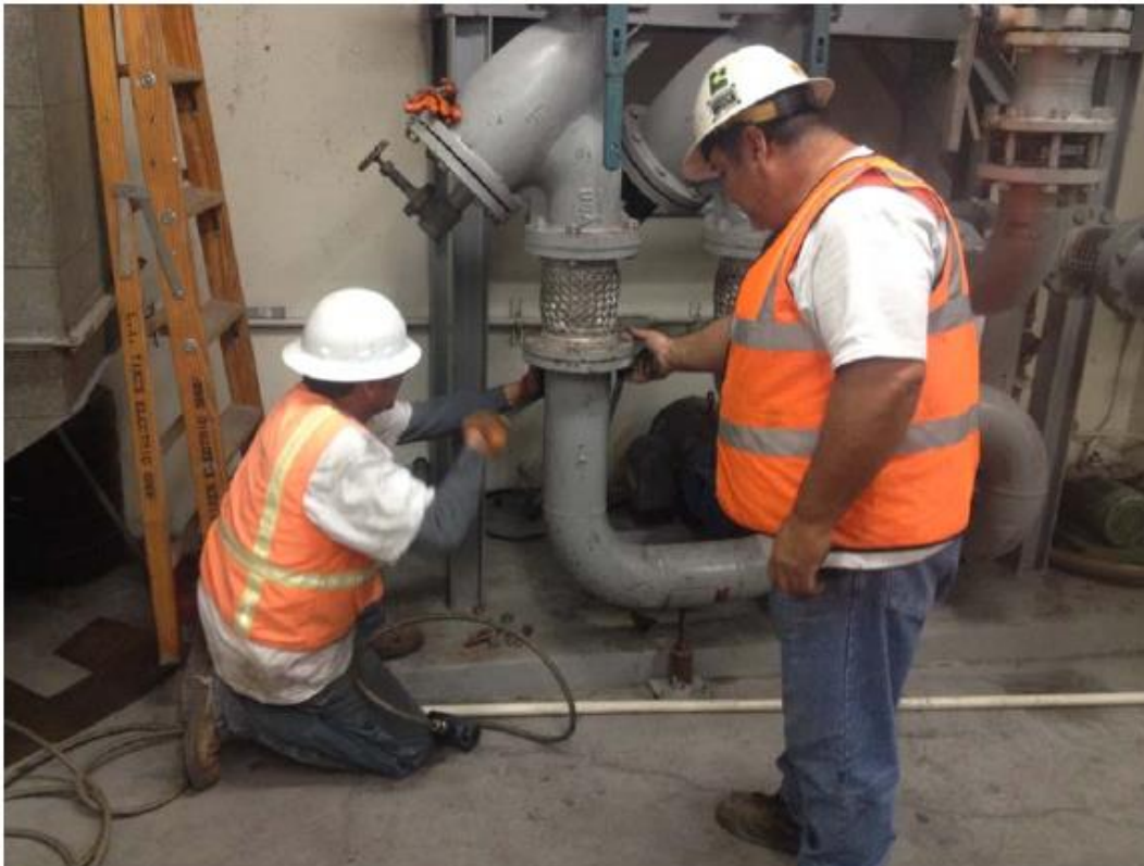
LA Times building basement piping removal
