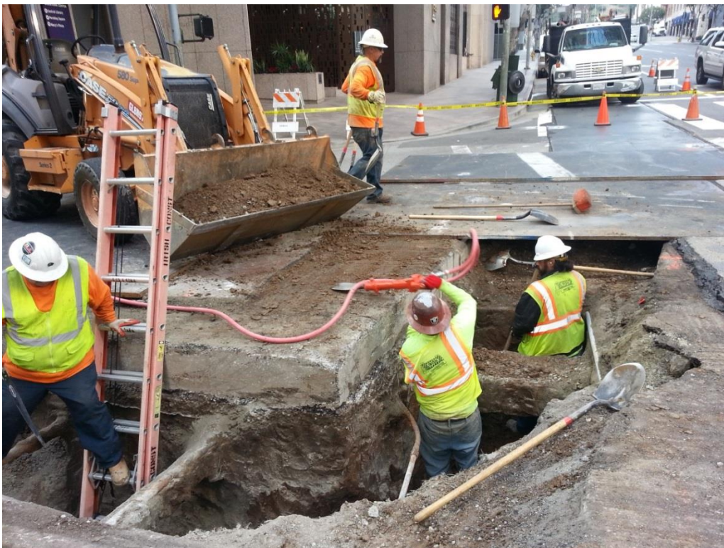
Sixth Street and Flower – Level 3 trench work by Irish Construction, Inc.
