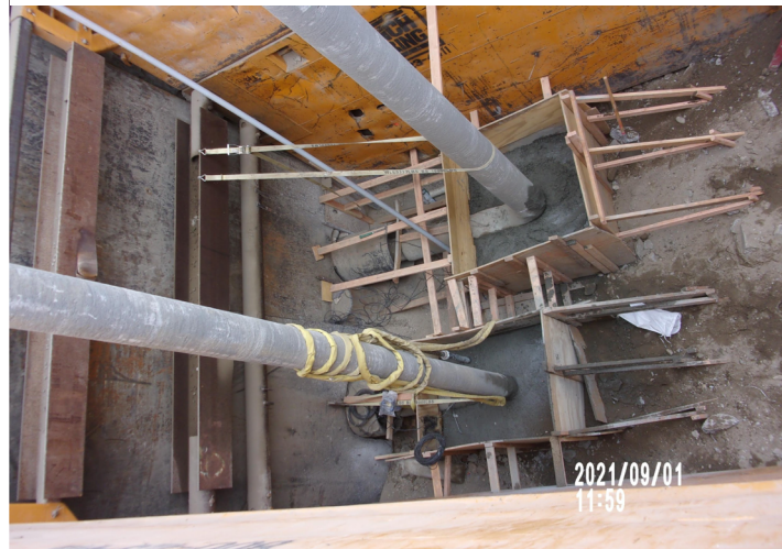
Micropile drilling for storm drain support and protection.
