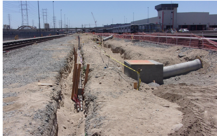
Installing lighting ductbank at Road A area.
