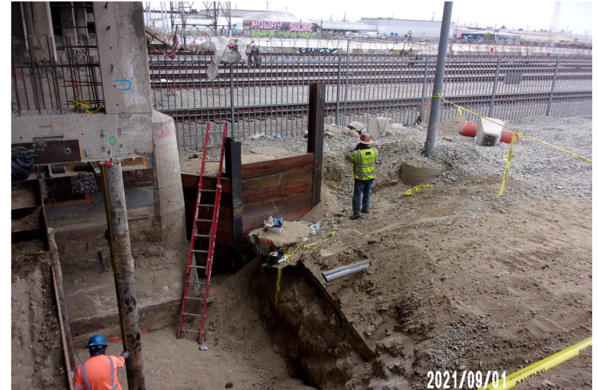
Bracing the bridge in preparation of footing and wall additions at bent 12.
