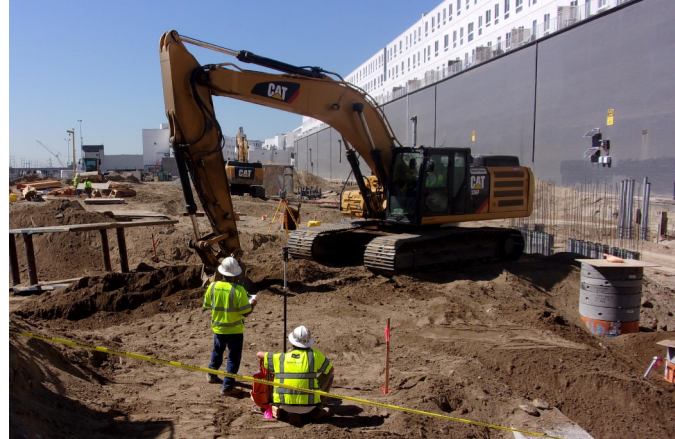
Ongoing excavation for ductbank installation for the new TPSS.
