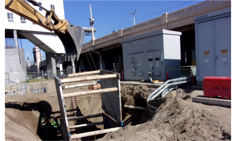
Installing a shoring box for ductbank excavation and protection.
