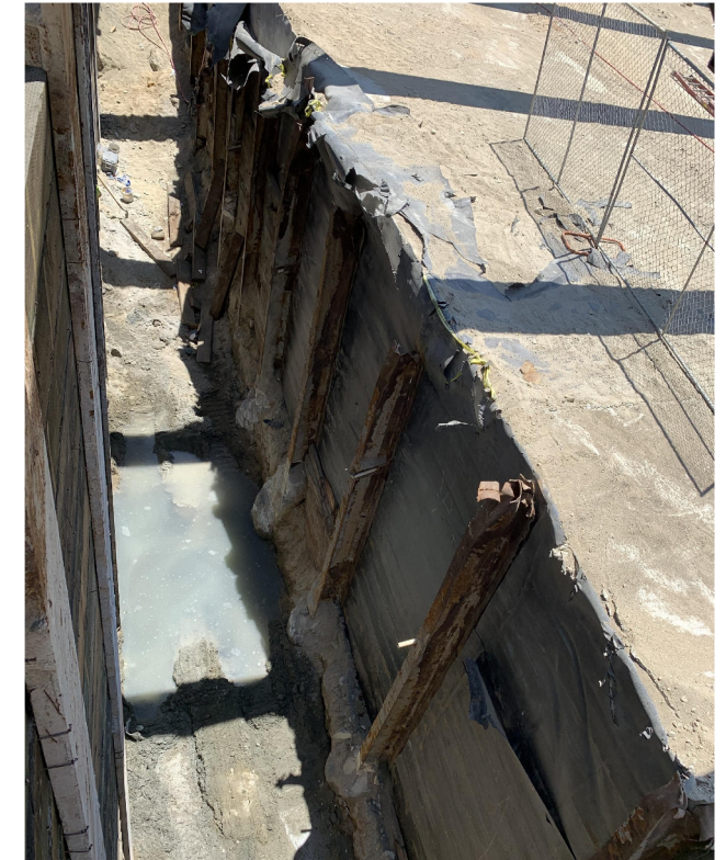
East wall for widened portal.
