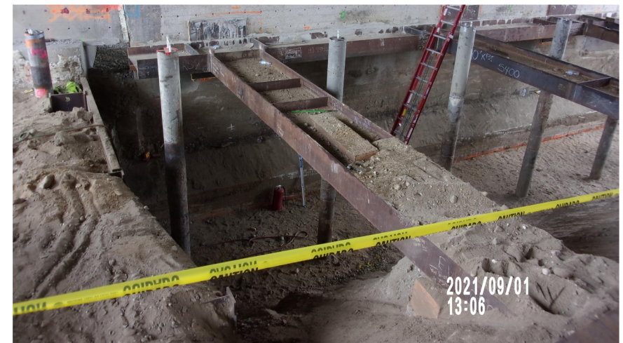
Bracing the bridge in preparation of footing and wall additions at bent 12.
