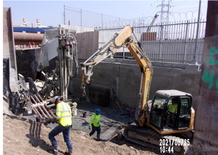
Micropile drilling for storm drain support and protection.
