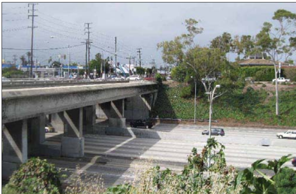
Exhibit 1. Florence Avenue/I-405 Railroad Bridge, looking west.
