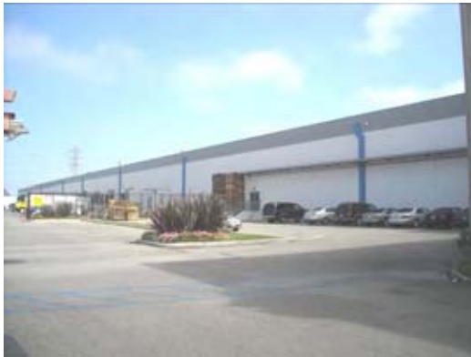
Figure 3-20. View of industrial warehouse on the site
