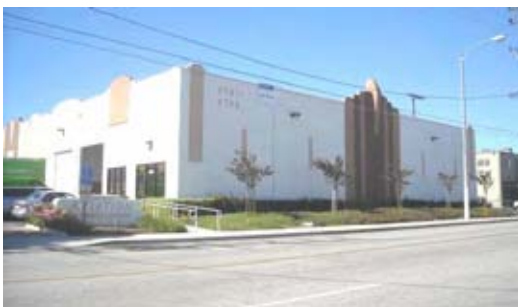
Figure 3-18. View of Aviation Business Center on the northern end of the site
