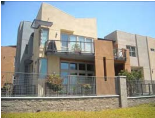
Figure 3-26. View of multi-family residences to the south of the site.
