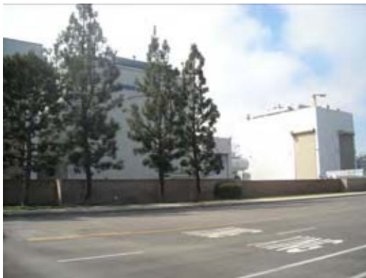
Figure 3-22. View of industrial uses to the west of the site
