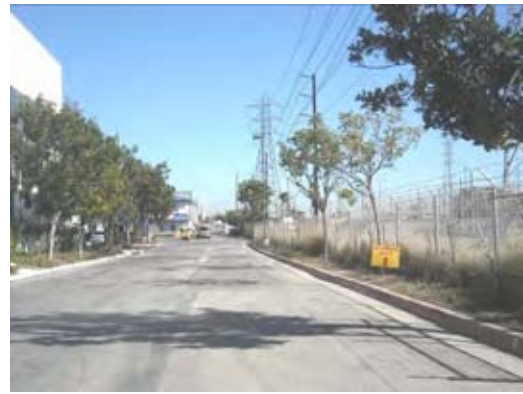
Figure 3-27. View of utility easement to the south of the public storage facility.
