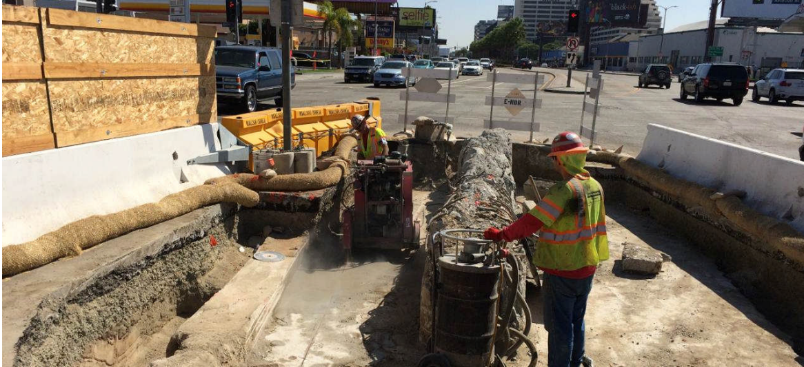
Saw cutting the existing Aviation bridge center bent footing.
