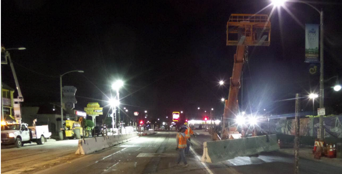
Relocating k-rails from east side to west side of Crenshaw.
