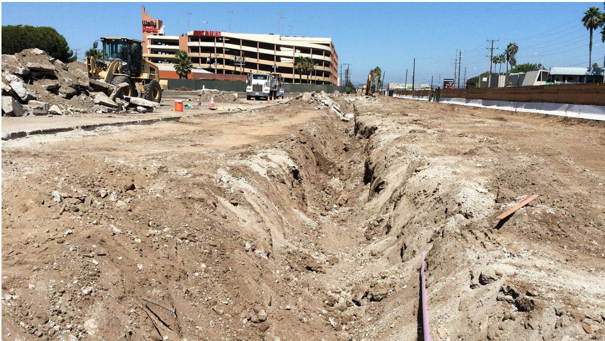
Wally Park Yard Storm Drain Removal Trench.
