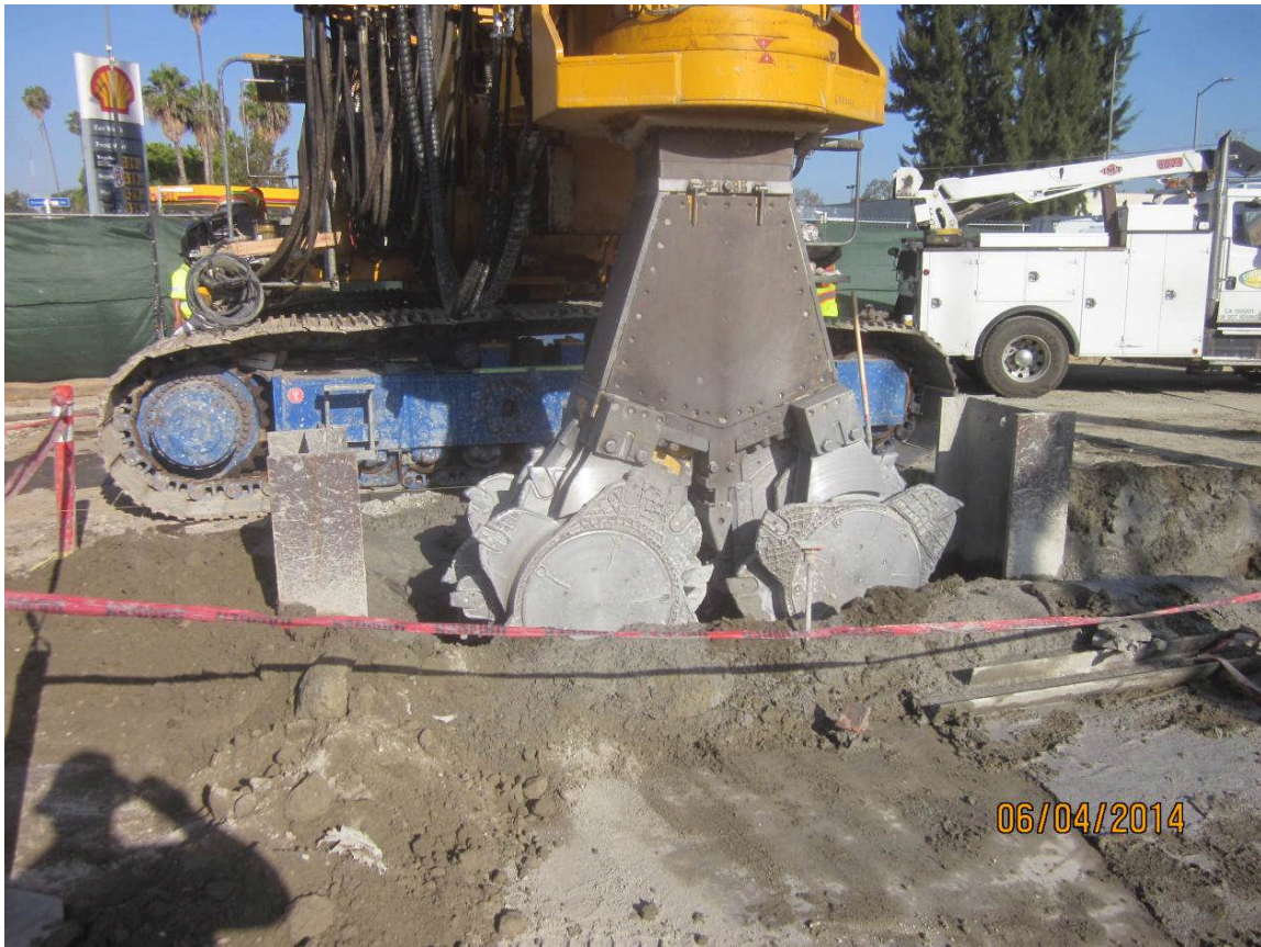
Cutter soil mixing equipment at the Exposition Station Yard.
