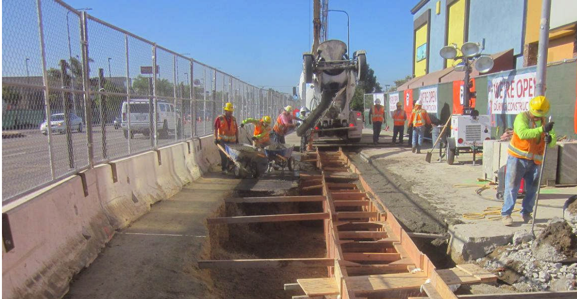
Support of excavation trench on Crenshaw Boulevard (west).
