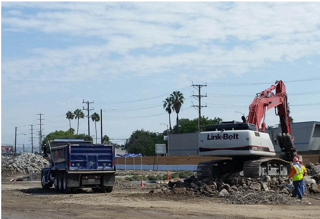
Century Bridge demolition material processing and haul out.
