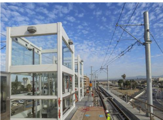
Aviation/Century Station elevator progress
