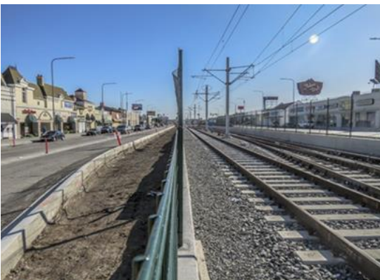
Park Mesa Heights light rail guideway fencing Crenshaw Bl.
