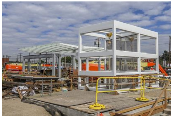
Leimert Park Station plaza glass canopy and elevator structure
