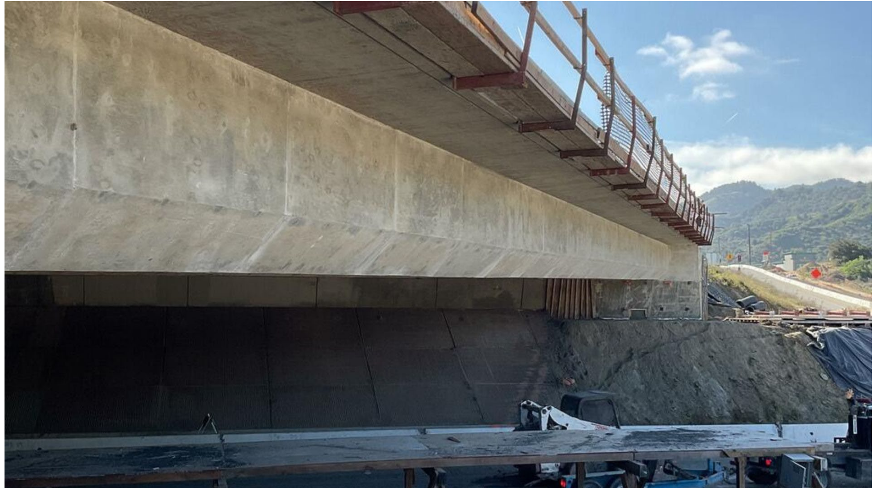
Calgrove BI Undercrossing bridge, April 2024
