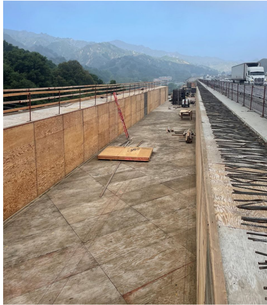
Falsework installation at Gavin Canyon Bridge, March 2024
