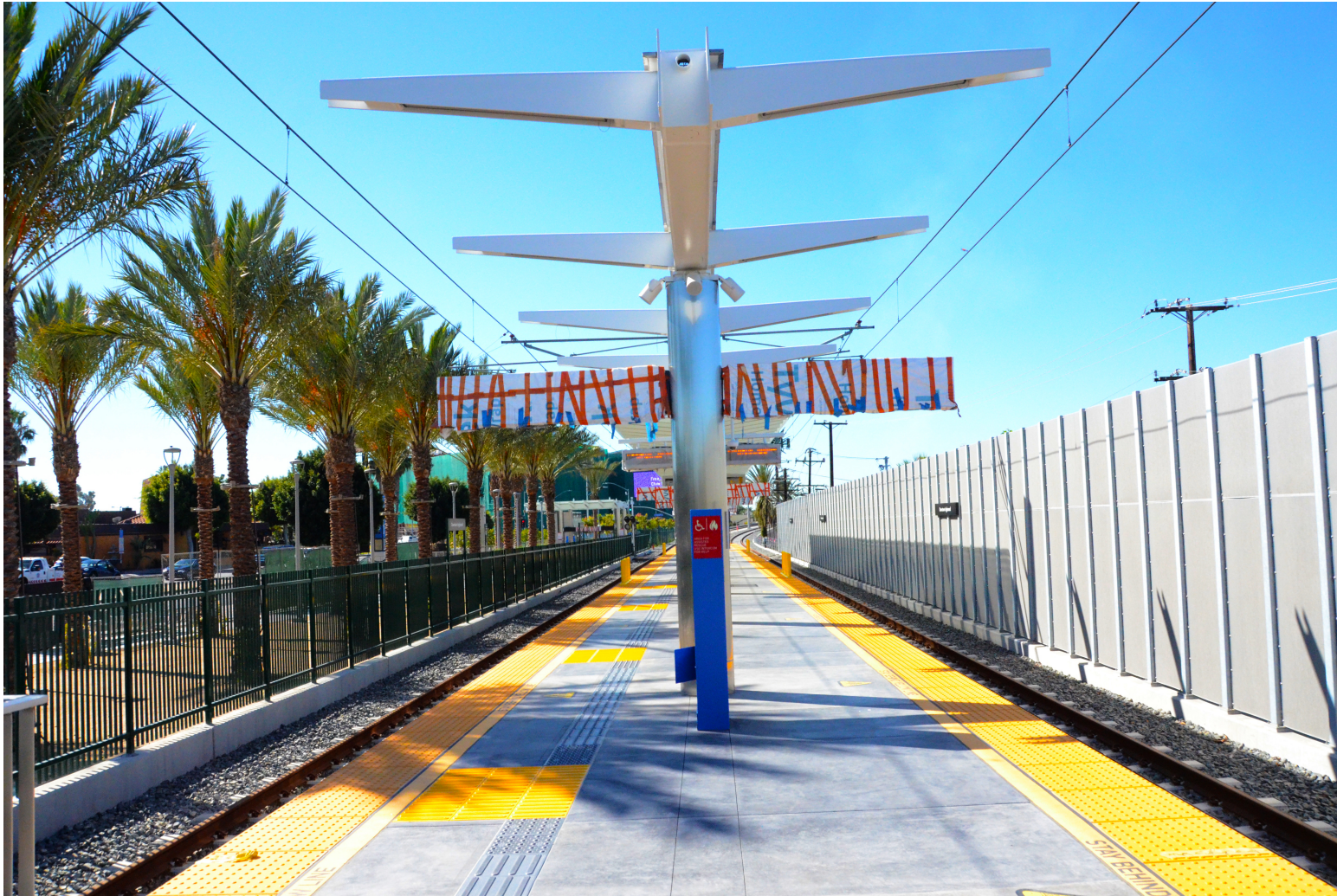
Station platform installed signage and yellow tactile pavers
