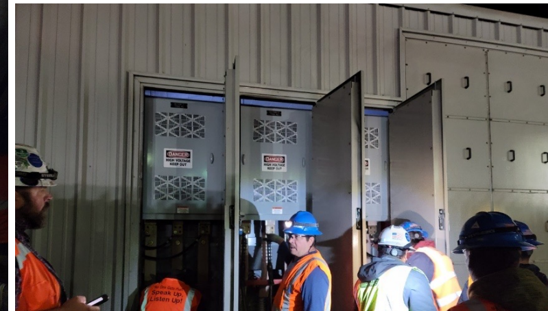
Resolving remaining work items for TPSS
