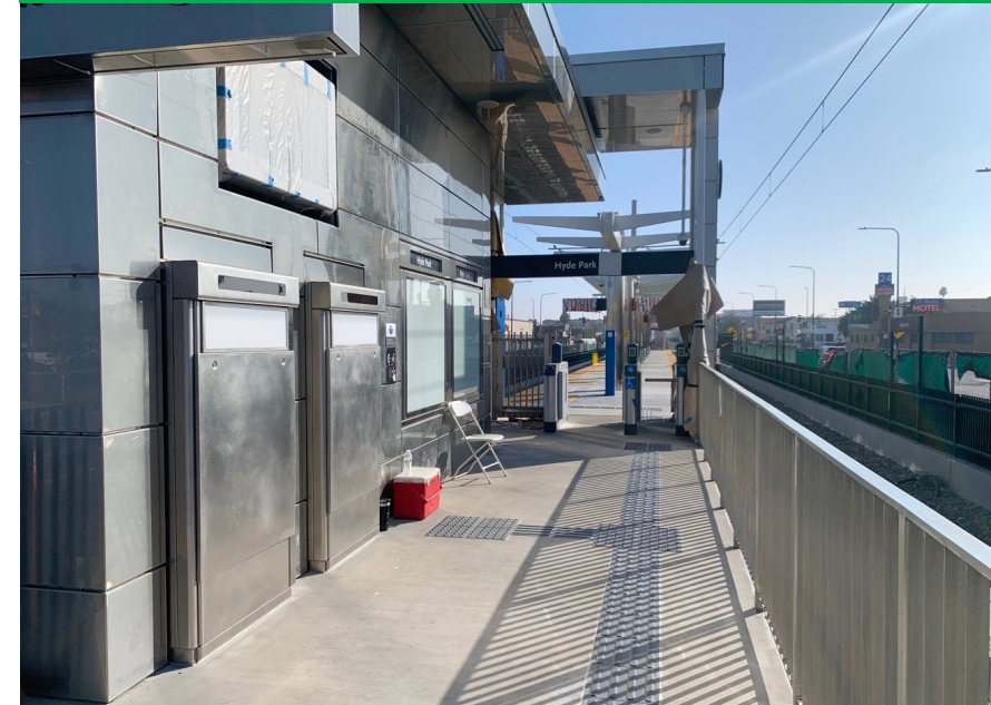
Installed TVM and map casings
