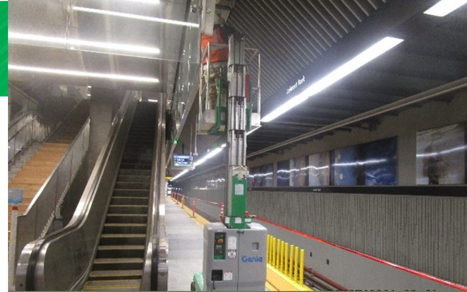
Installing drop ceiling trim panels around the smoke screen glass perimeter
