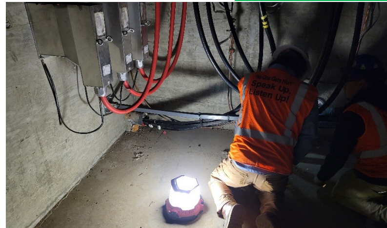
Remaining items Remedial work for TPSS #2 Vault
