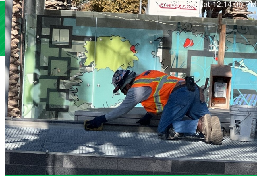
Grouting tile for the fresh air intake shaft at the plaza
