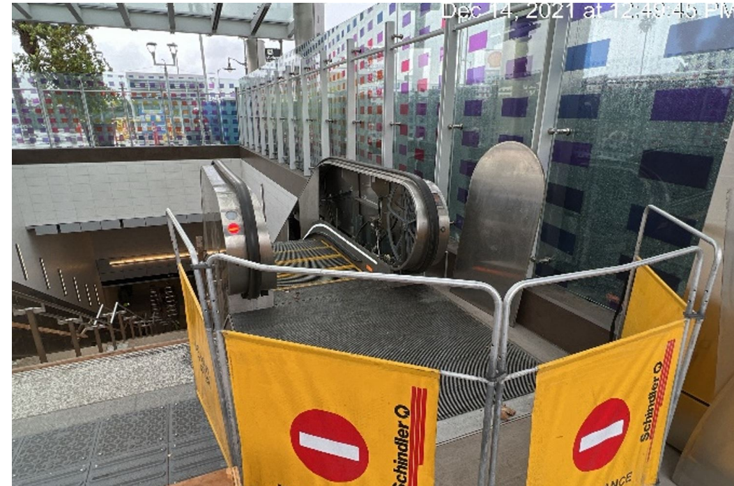
Performing operation testing of escalator at the main entrance
