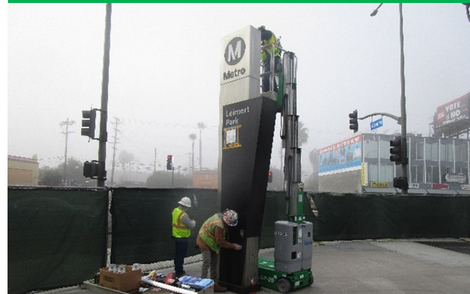
Cleaning and polishing the grand pylon sign at the plaza
