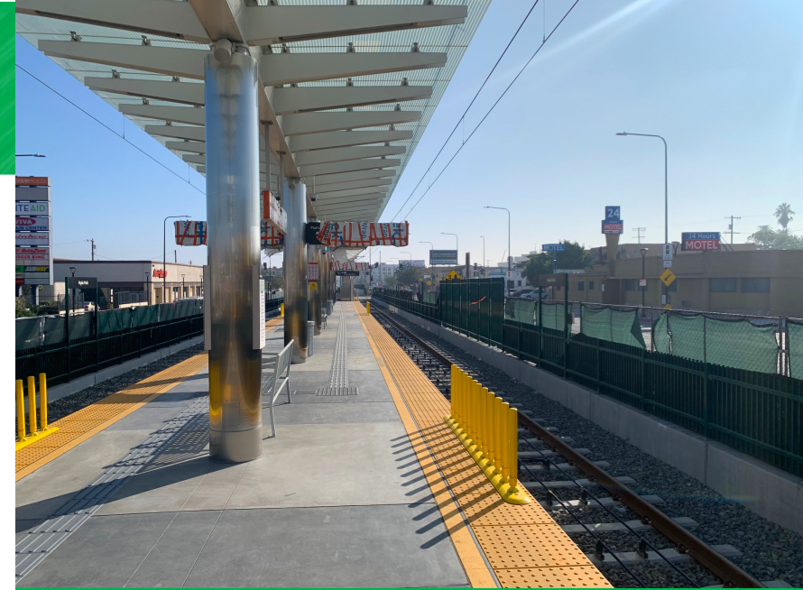
Station platform and tactile pavers
