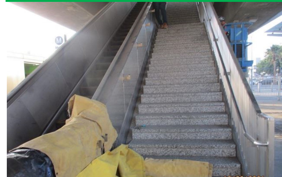
Mounting handrailing on the inside of the stairways
