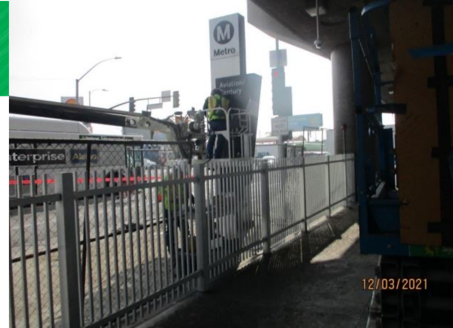
Applying signage for the grand pylon
