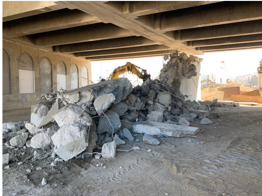
Bent 16 demolition continues.
