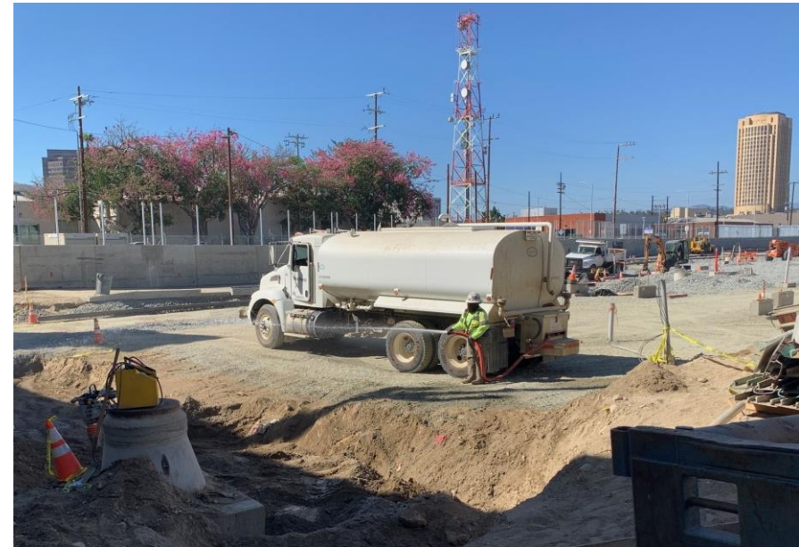
Contractor team supporting the backfill operation with dust mitigation.
