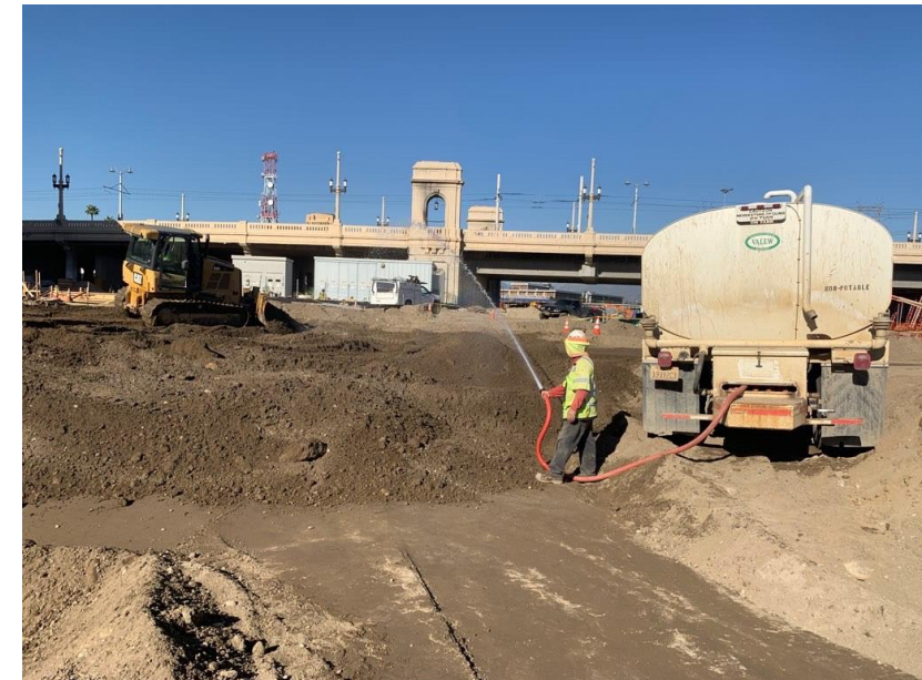
Contractor team supporting dust mitigation in the south yard.
