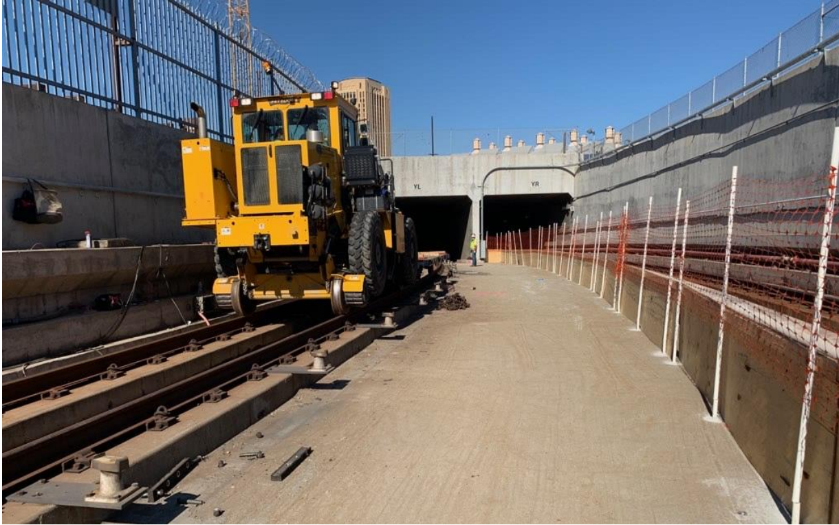
Equipment beginning demolition of tracks south of the portal.
