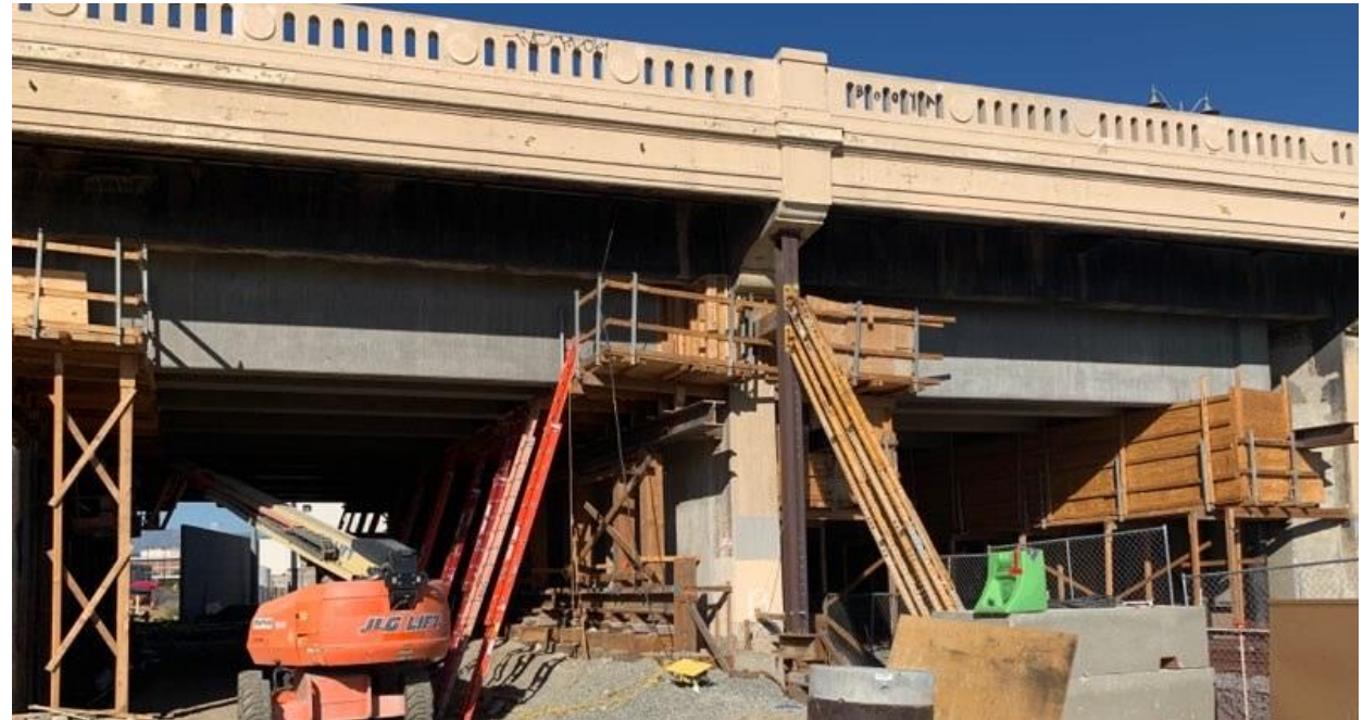
Girders installed on to support the removal of Bent 13.
