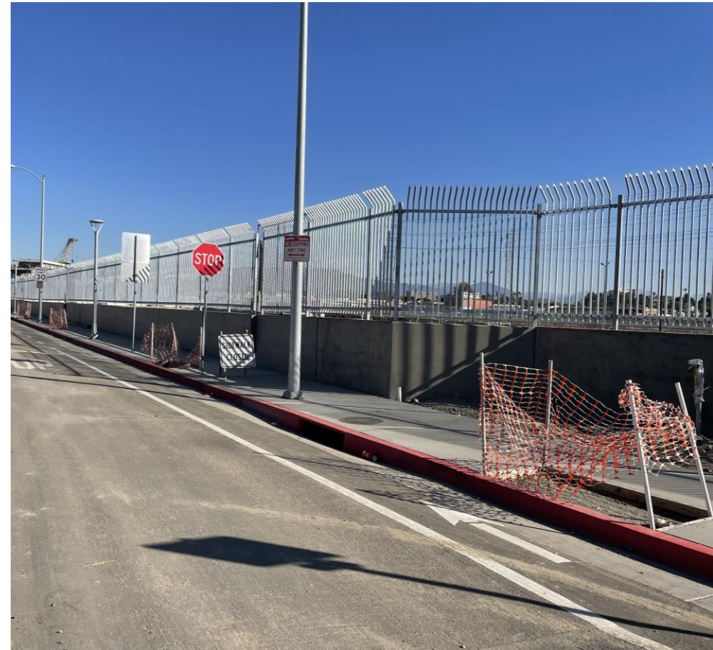
The permanent fence and lighting installed above.
