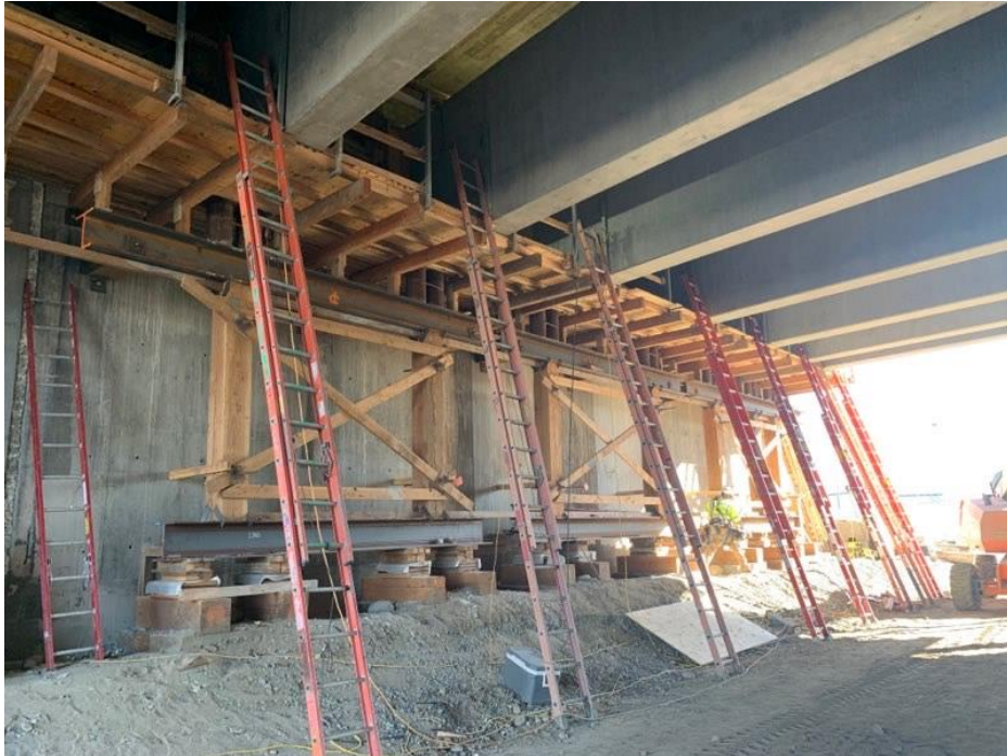
Falsework and bracing for the bent support at Bent 13.
