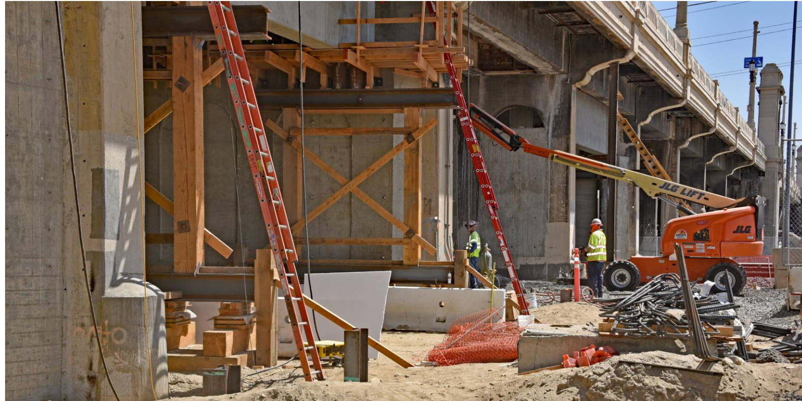
Complicated work on the south end of 1st Street Bridge.
