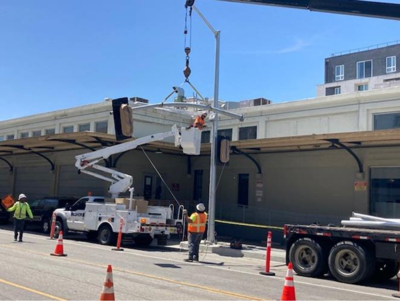
Mid-block Crossing on Santa Fe Av between 3rd and 4th St
