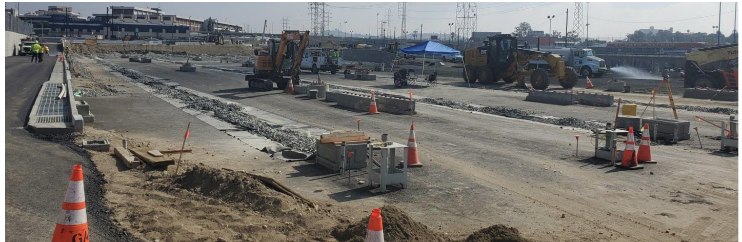
Access roads and drains have been added to the north yard.
