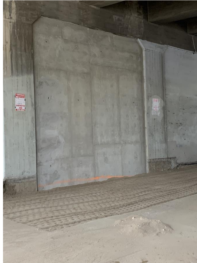
Here is an example of a completed wall infill.
