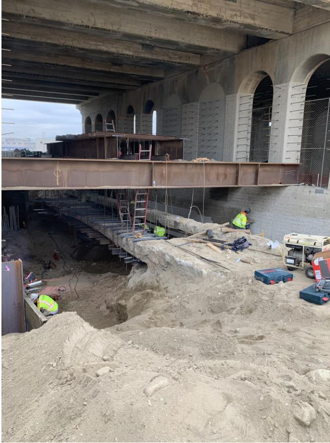
1st Street Bridge bracing and other concrete repair continues.
