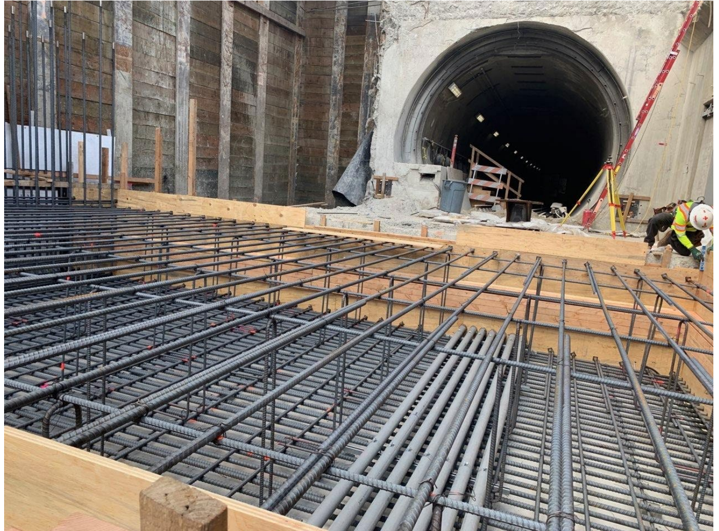
Preparation for concrete slab pour on the tunnel's west side.
