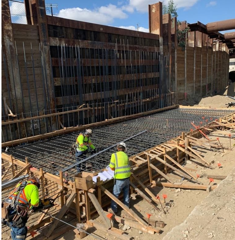
Storm drain protection in the west portal area.
