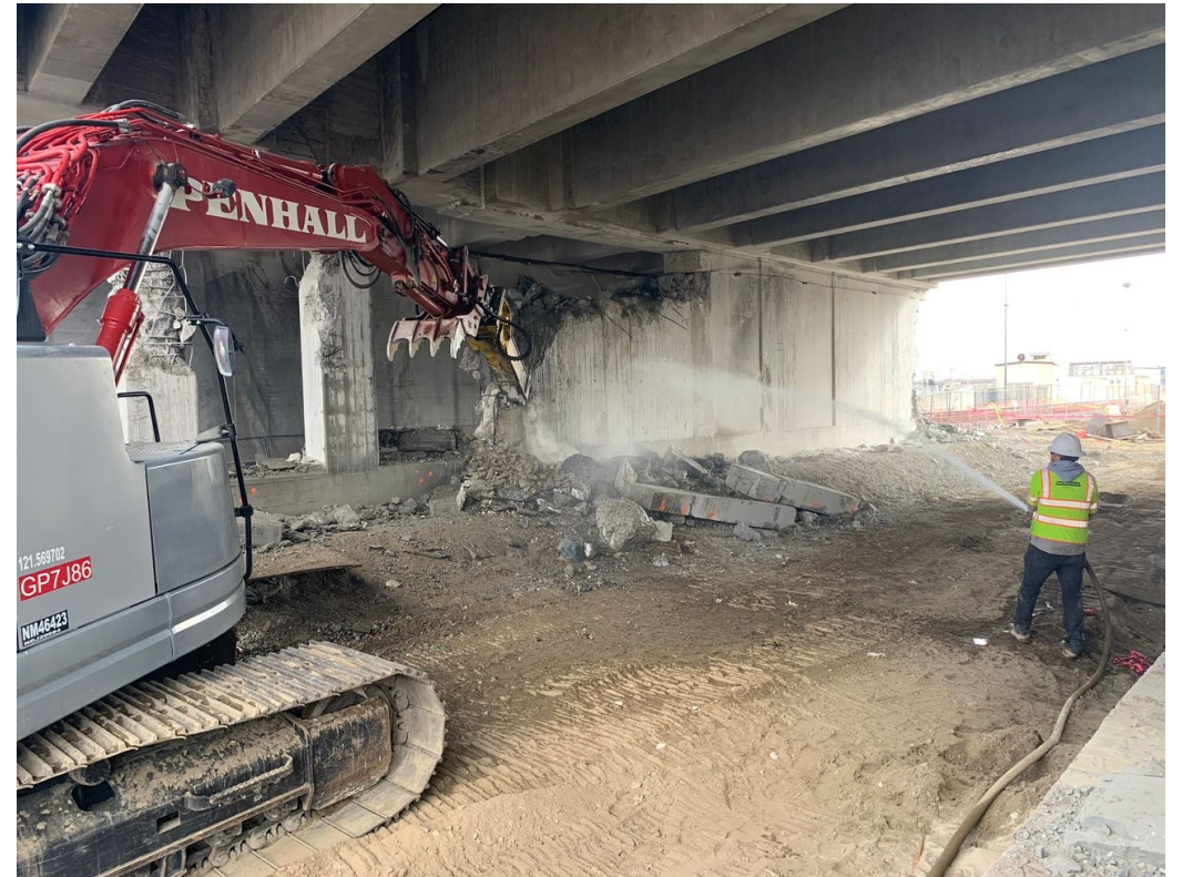
Workers support dust mitigation during Bent 13 demolition.
