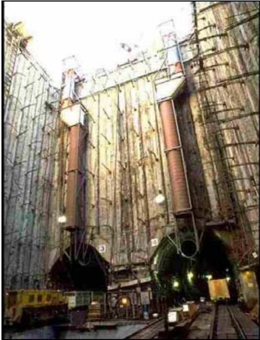
SECANT PILE WALLS, BARNSDALL SHAFT, HOLLYWOOD
