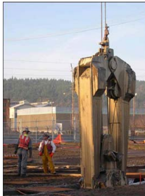
SLURRY WALL EXCAVATION, PORTLAND, OR
