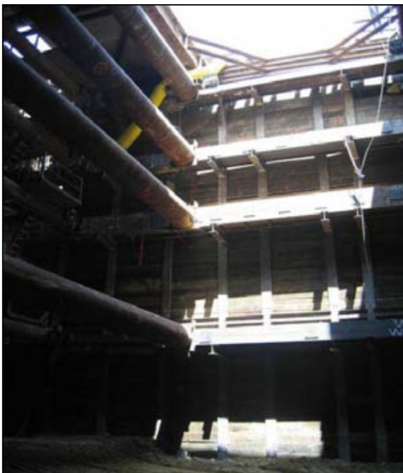
SOLDIER PILES AND LAGGING WITH CROSS BRACING, MARIACHI PLAZA, MGLEE
