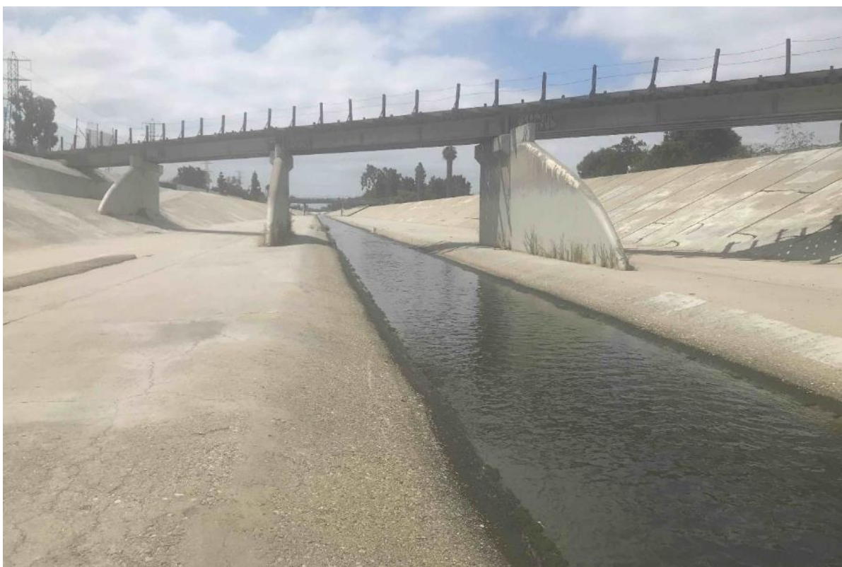
Photograph 8. Low flow channel within San Gabriel River, facing south.
