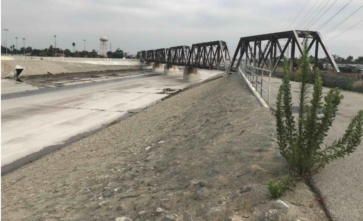
Photograph 1. Los Angeles River, facing north.
