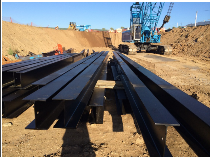
Soldier Beams at Azusa-Citrus Parking Structure
