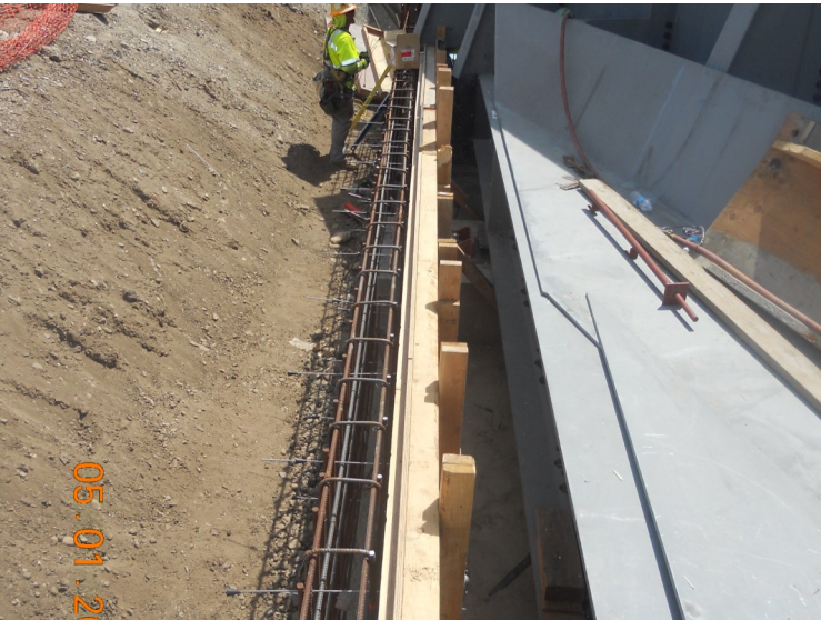
Segment 4: Foothill Bridge - Backwall Construction
