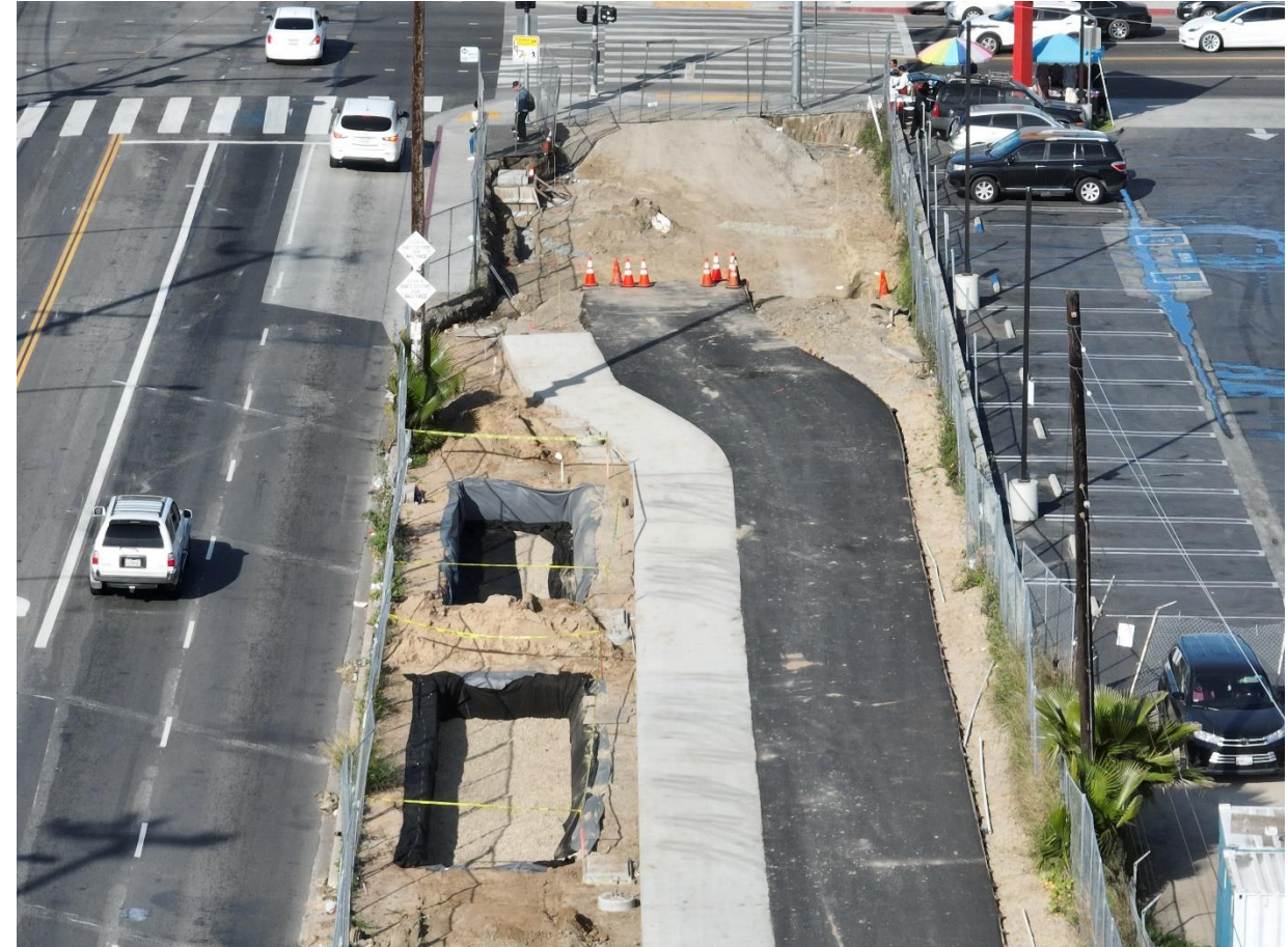
Field crew placed gravel in BMPs
