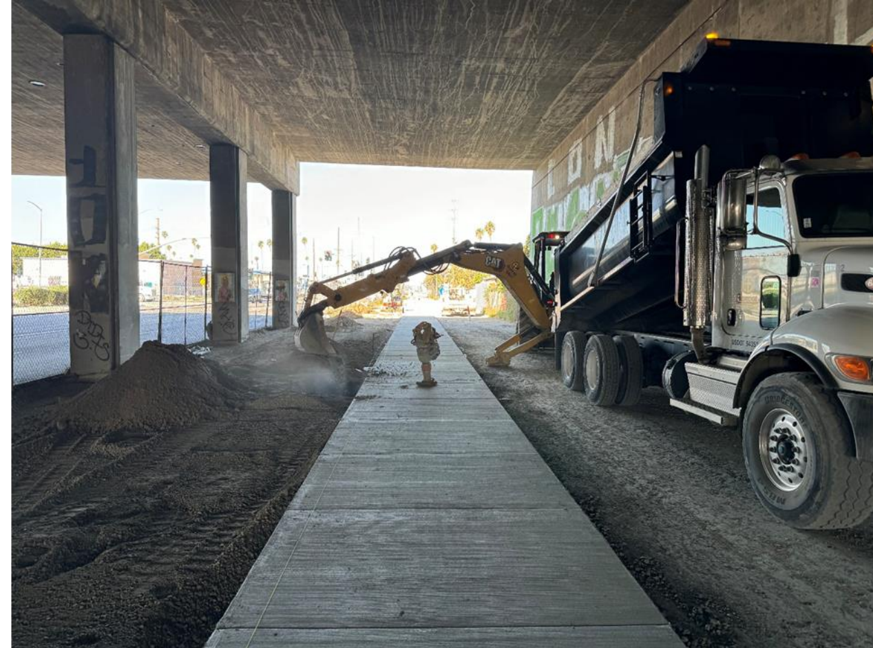
Metro Right of Way under the 110 FWY west view
