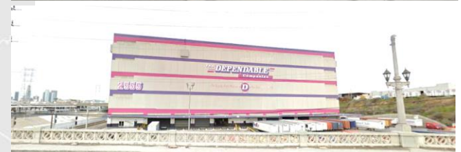
B. Distribution Center
