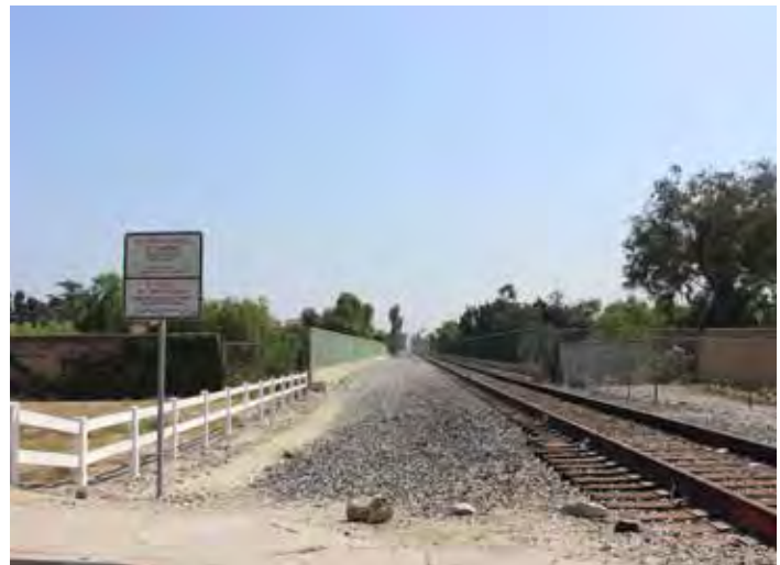
Existing rail alignment across the I-105 Freeway
