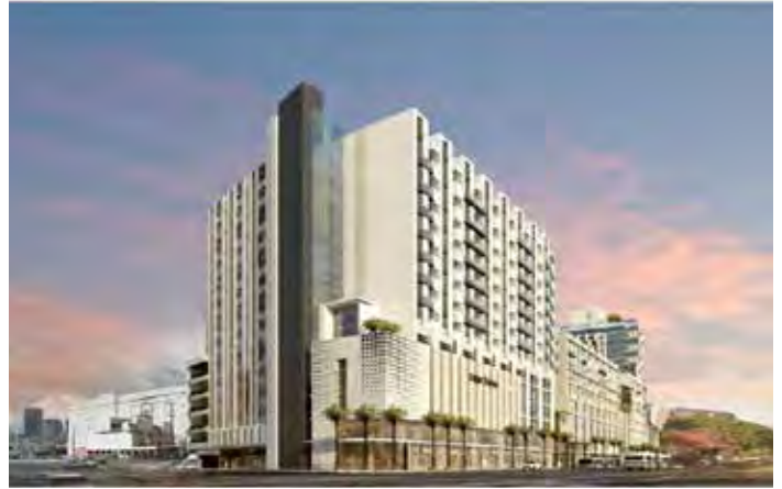
Little Tokyo Galleria Development
