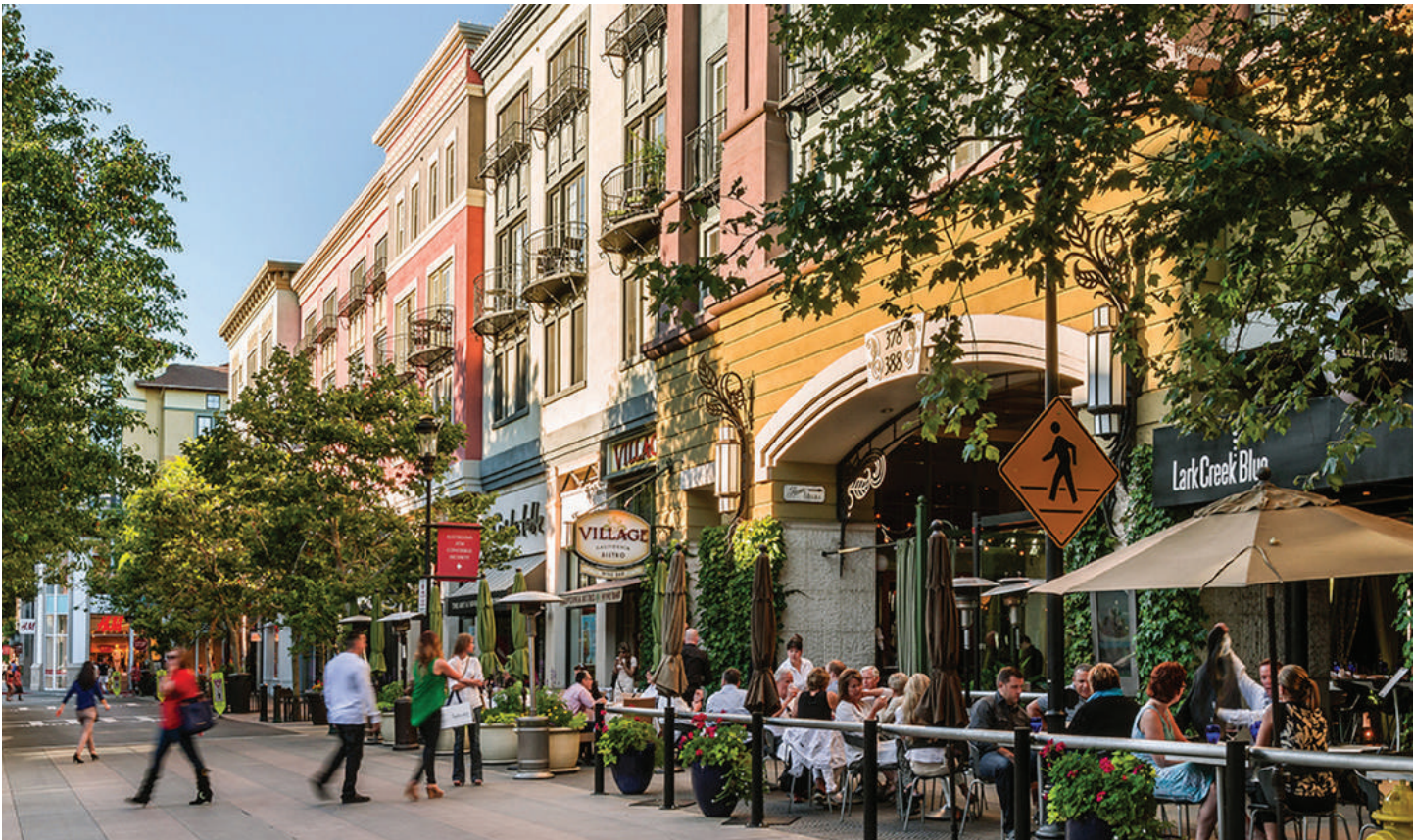
Santana Row mixed-use development in San Jose was identified as a precedent for development in the station-area.
