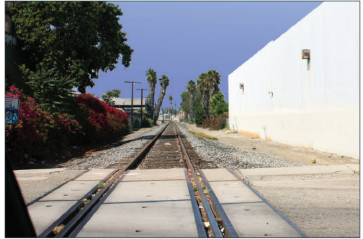
Existing Conditions , I-105/Green Line Station
