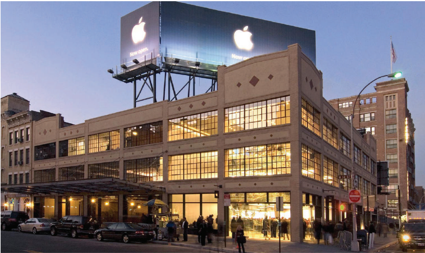
Adaptive reuse of unique industrial buildings for light industrial or commercial office uses should be considered.
