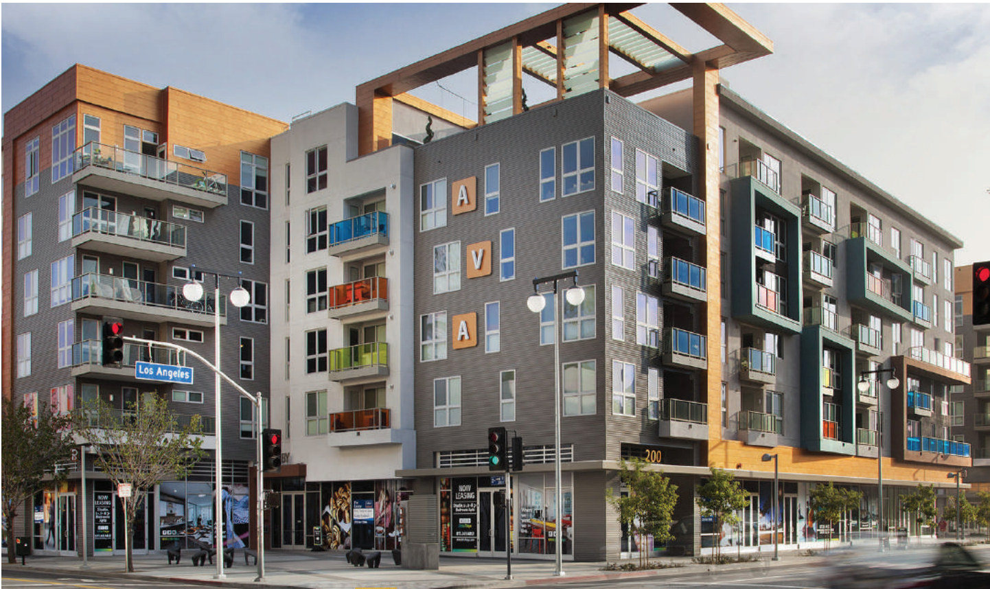
High density residential mixed use with active ground floor uses that activate the public realm
