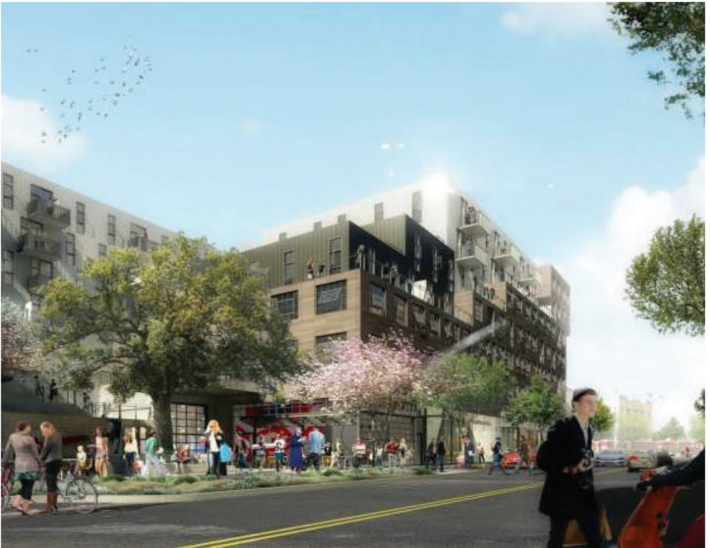
High density residential mixed-use that has active ground level uses creating a vibrant public realm
