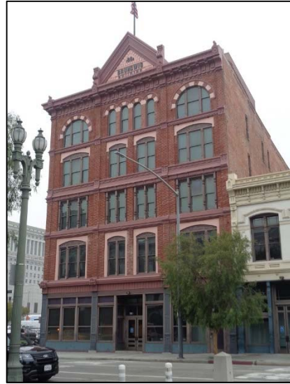
Figure 6: Vickrey-Brunswick Building, camera facing west. ICF, 2018.
