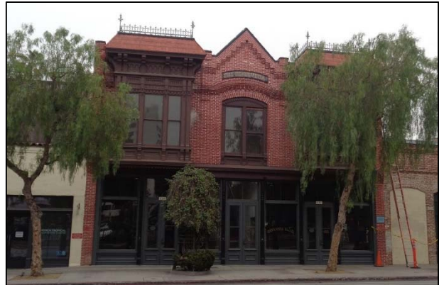
Figure 26: Sepulveda House, camera facing southeast. ICF, 2018.
