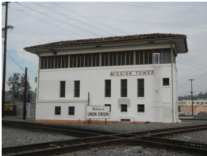
Looking north, Photo #DSCN2985.jpg Photo: ICF International, 1/9/2015
