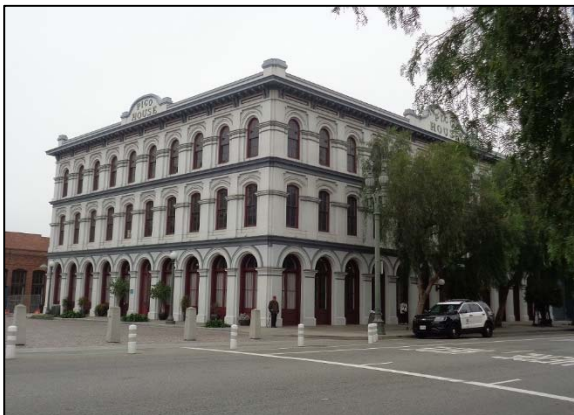
Figure 7: Pico House, camera facing south. ICF, 2018.
