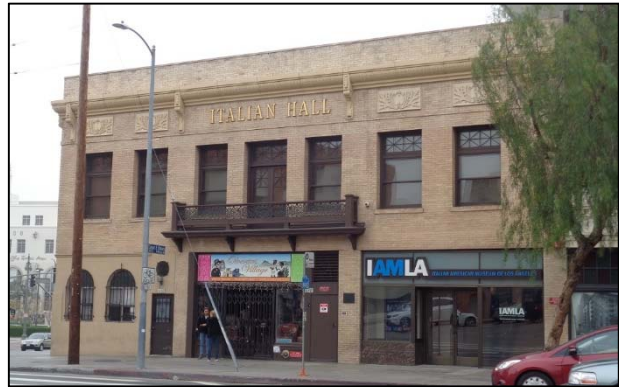
Figure 22: Italian Hall, camera facing east. ICF, 2018.
