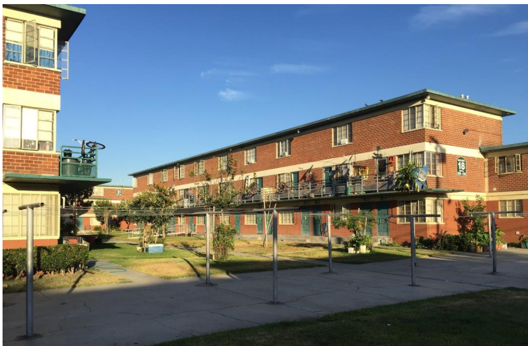
William Mead Homes apartment building. Camera facing southwest. ICF International, 11/7/2014
