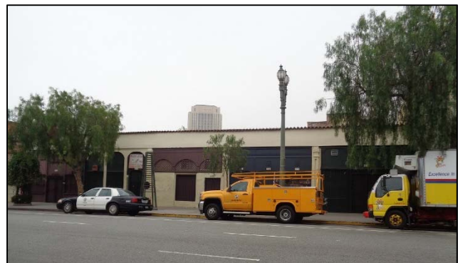
Figure 28: Jones Building, camera facing southeast. ICF, 2018.
