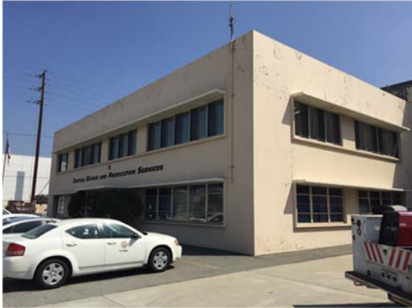
Building 16: Administration Building, 1957, (19-176371). Camera Facing NW. Photo ICF International, July, 2016. IMG_9073.jpg
