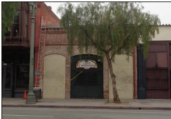
Figure 27: Machine Shop, camera facing southeast. ICF, 2018.
