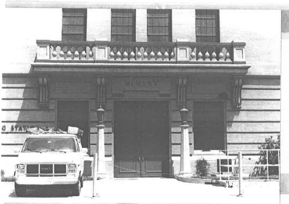
Building No. 5 (detail of entrance)-SE - Contributing
