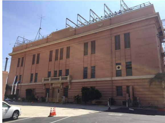
Building 5: Receiving Station A, 1925. (19-175283). Camera facing NE. Photo ICF International, July, 2016. IMG_9182.jpg
