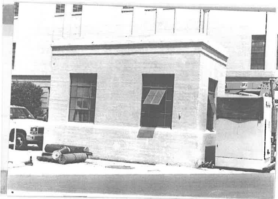
Hoist House-NE - Contributing
