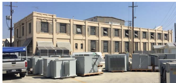
Building 11: Transformer Warehouse (Train & Williams, Architects), 1926. (19-175281) Photo: ICF International, July, 2016. IMG_9095.jpg
