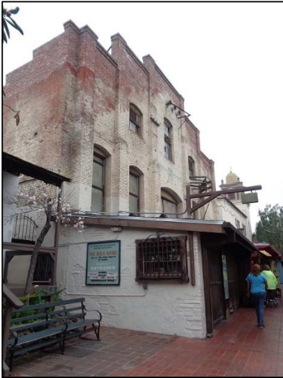
Figure 17: Plaza Substation, Olvera Street elevation, camera facing south. ICF, 2018.
