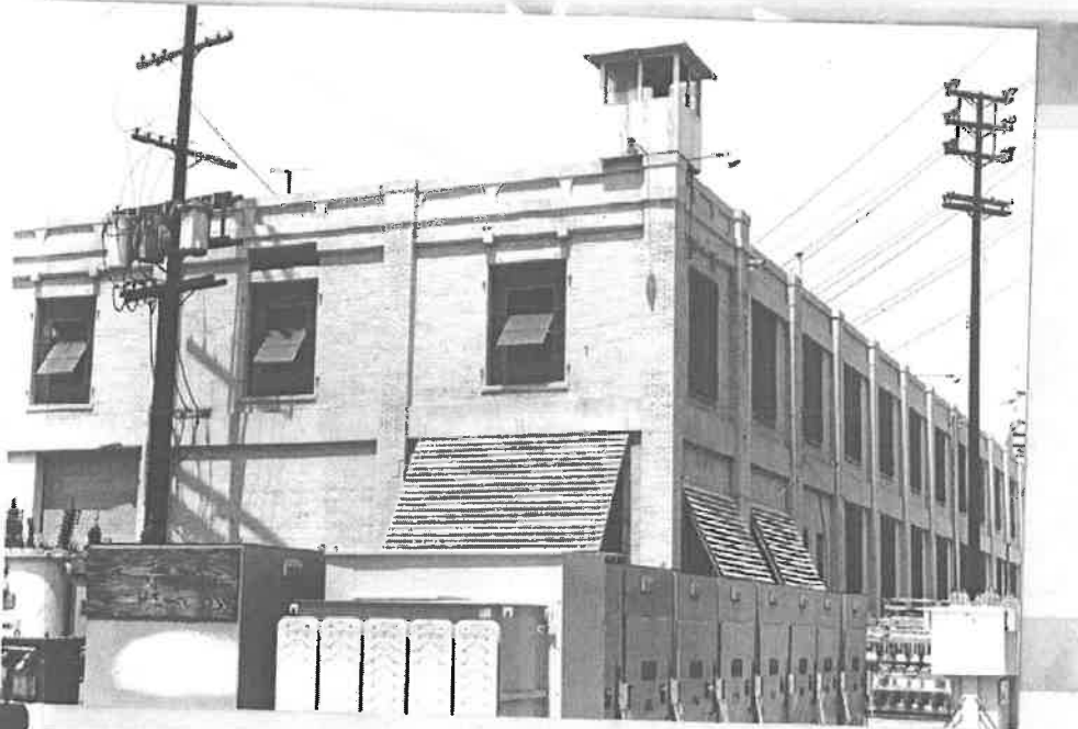
Building No. 11-E - Contributing
