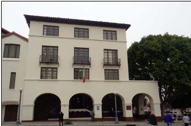
Figure 15: Biscailuz Building, camera facing northeast. ICF, 2018.
