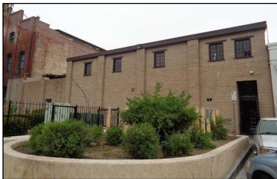
Figure 19: Avila Annex, camera facing northwest. ICF, 2018.
