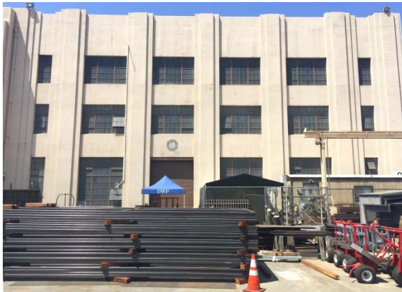
Building 9: Electrical Repair Shop, 1935/1937. (19-175284). Camera Facing S. Photo: ICF International, July, 2016. IMG_9276.jpg
