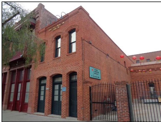
Figure 11: Sanchez Building, camera facing northwest. ICF, 2018.
