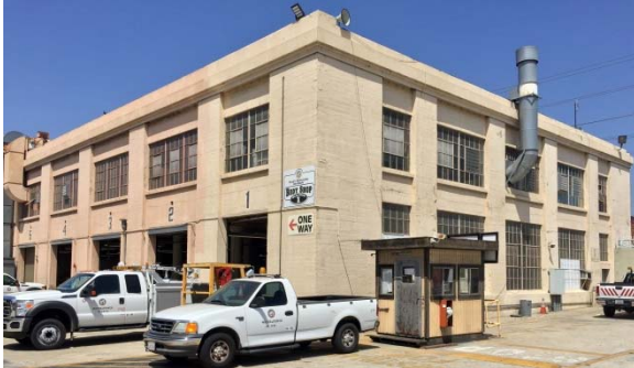
Building 1: Light Mechanical Shops, 1924. (19-175280). Camera Facing SW. Photo ICF International, July, 2016. IMG_9325.jpg
