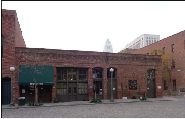
Figure 13: Hellman-Quon Building, camera facing south. ICF, 2018.
