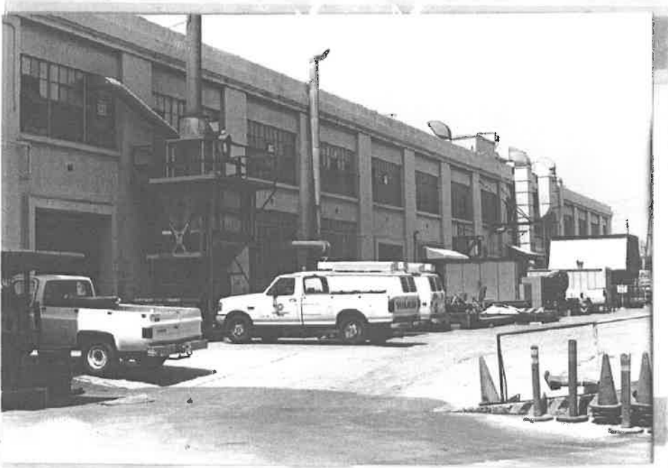
Building No. 1-NE - Contributing
