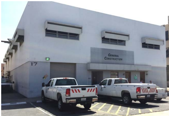
Building 17: Station Maintenance Building, 1963, (19-176373). Camera Facing SW. Photo: ICF International, July, 2016. IMG_9076.jpg
