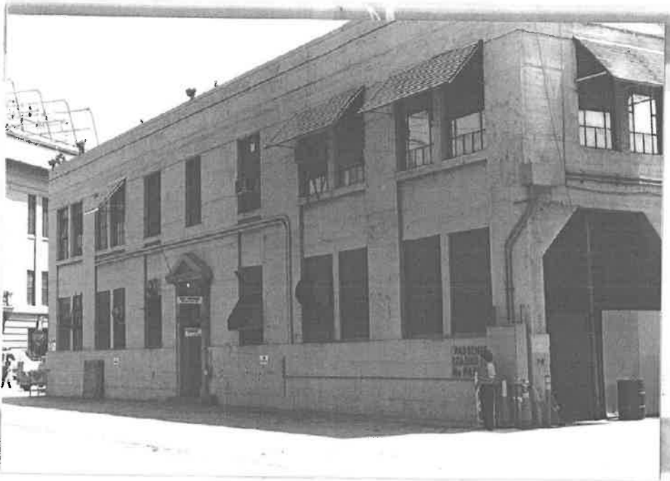
Building No. 3-W - Contributing
