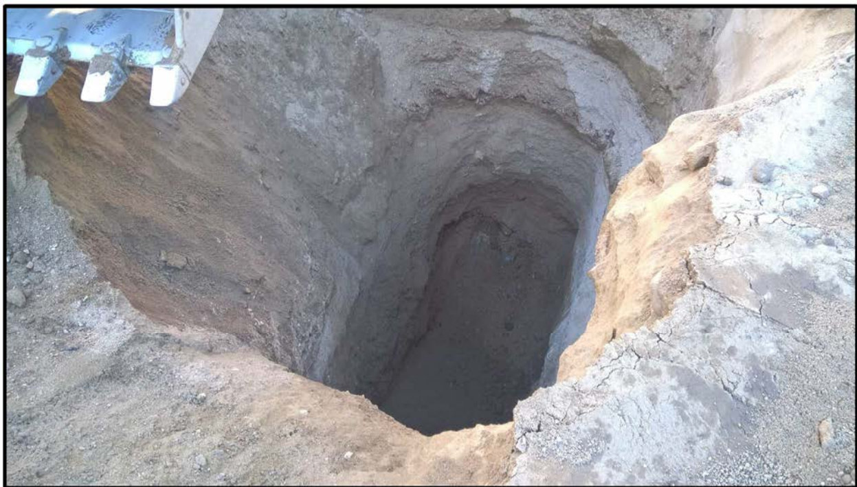
Photograph 28 – View on December 18, 2015 looking at bottom of pothole excavated in floor of Excavation Area EA-5 to approximately 34 feet below ground surface.
