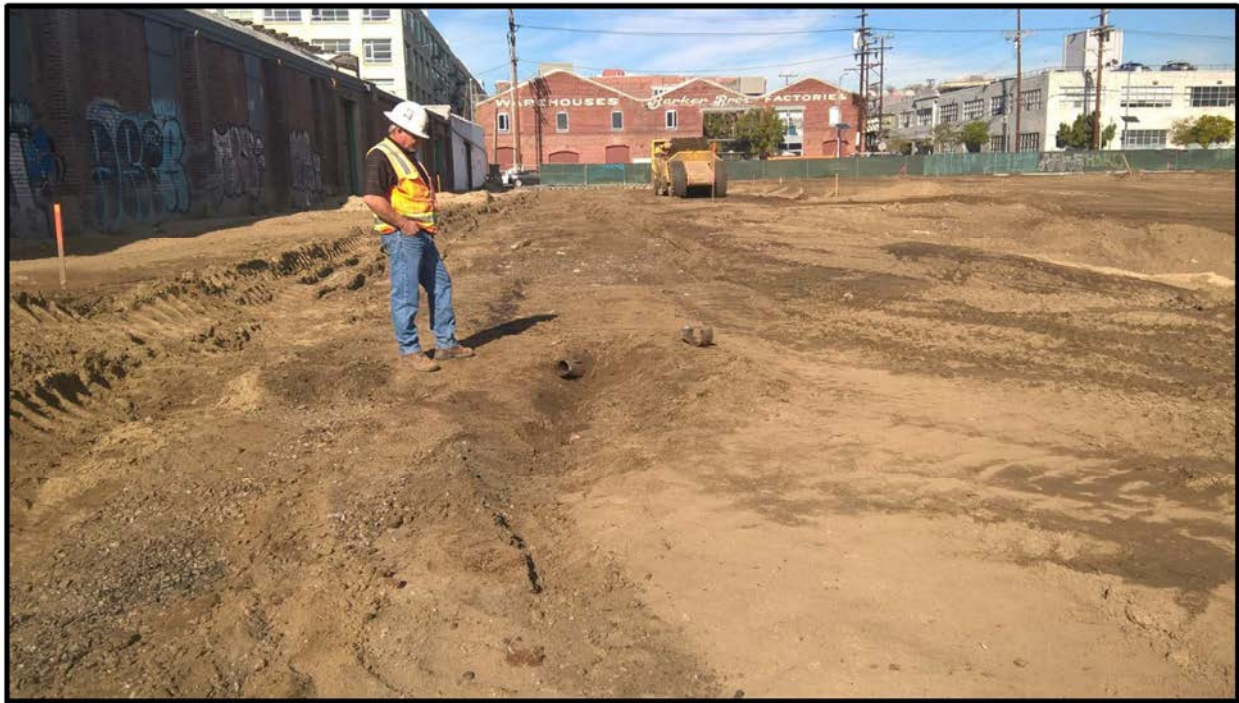
Photograph 19 – View on December 7, 2015 of old oil piping encountered near the Site surface.
