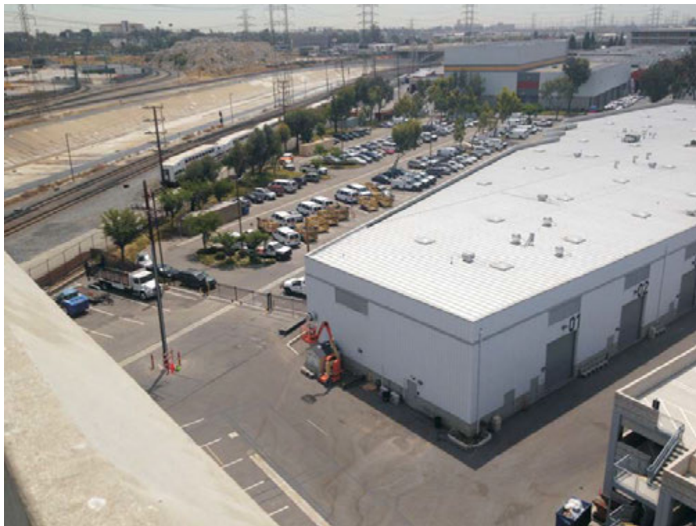
Looking south-east from top of parking structure
