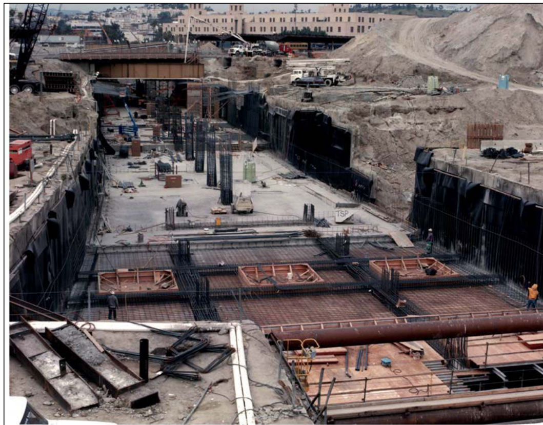
Photo No. 3. Mezzanine floor slab in place with column reinforcement steel protruding. The reinforcement for lift No. 4 of mezzanine floor is being placed in the foreground. Photo Taken: 01/30/90. Source: SCRTRD, 1990a.
