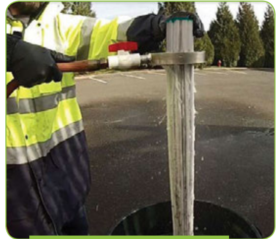
The Jellyfish Filter tentacle is light and easy to clean.
