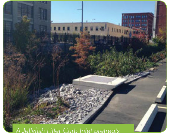
A Jellyfish Filter Curb Inlet pretreats runoff entering a bioretention system
