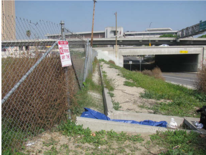
Photograph 7. Two-foot-wide drainage ditch along the fence line on the corner of Commercial and Center Streets, looking north
