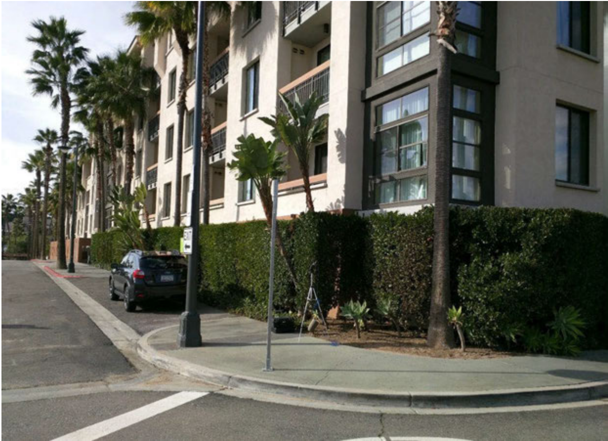
Figure 7-13. Monitoring Location 3 – Vibration Measurement at Mozaic Apartments
