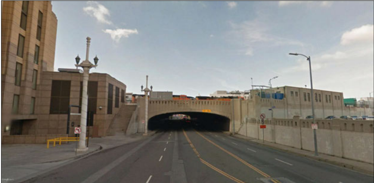
Figure 4-6. Key View #3a – Cesar Chavez Avenue (view looking west from road toward bridge)
