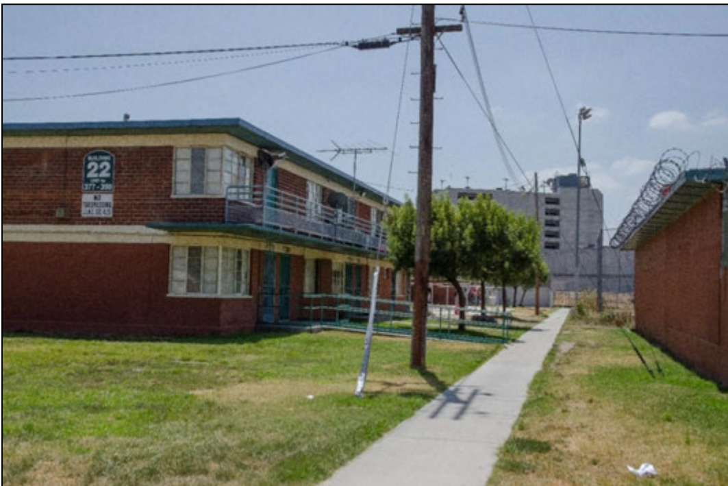
Figure 4-3. Key View #1b – William Mead Homes (view looking south from Elmira Street toward railroad right-of-way)
