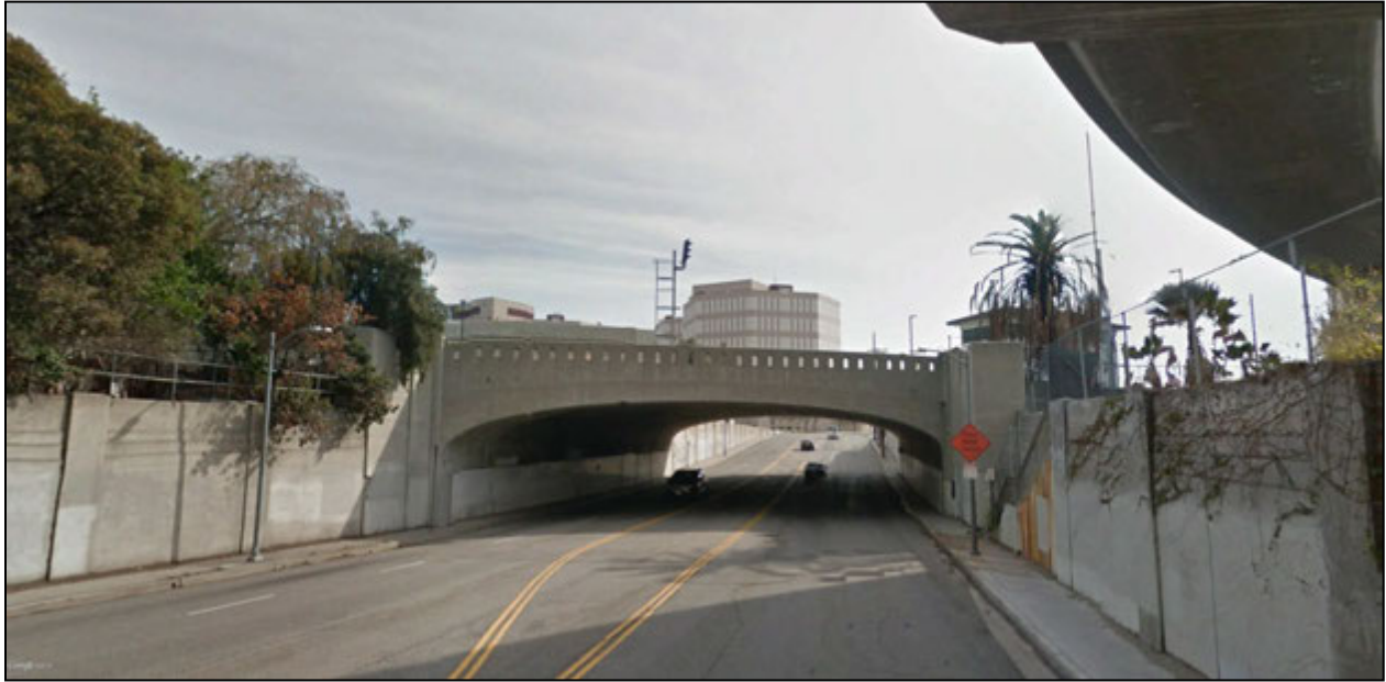
Figure 8-10. Key View #2b – Vignes Street Bridge (view looking east toward bridge) Existing Project Conditions
