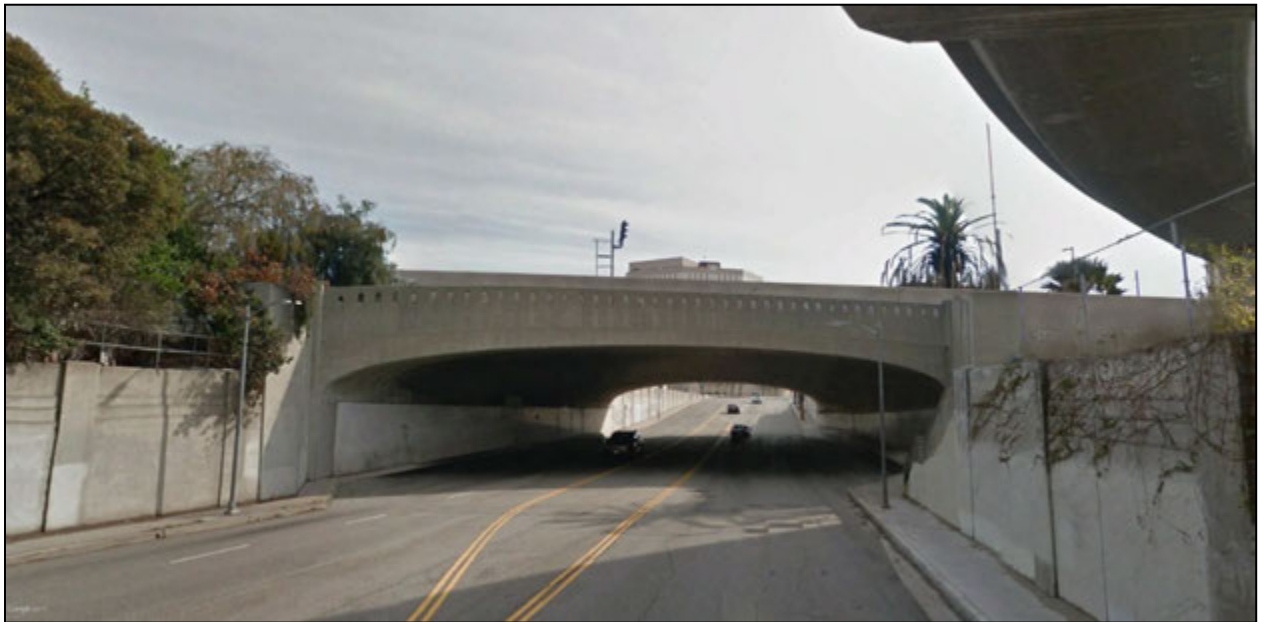
Figure 8-11. Key View #2b – Vignes Street Bridge (view looking east toward bridge) Post-Project Conditions
