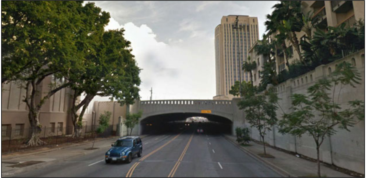
Figure 8-14. Key View #3b – Cesar Chavez Avenue Bridge (view looking east toward bridge) Existing Conditions
