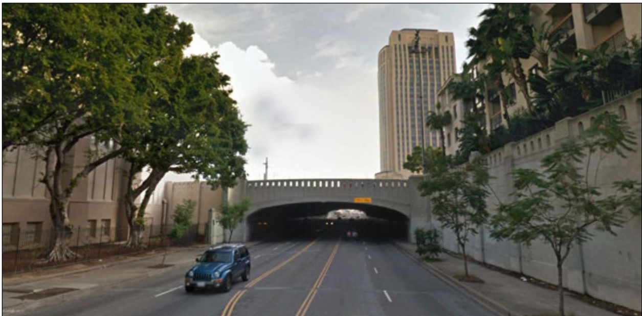
Figure 4-7. Key View #3b – Cesar Chavez Avenue (view looking east from road toward bridge)
