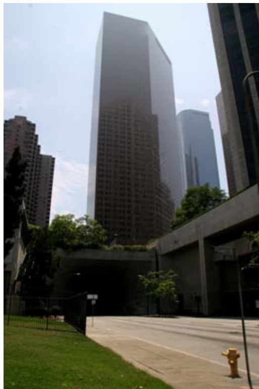
Figure 4-14. West End of 3 rd Street Tunnel
