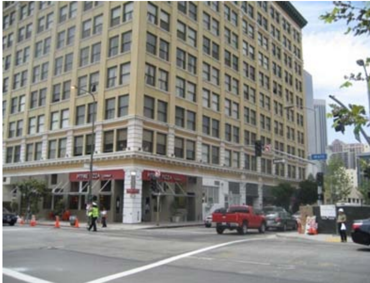
Figure 4-18. 2 nd Street and the Higgins Building
