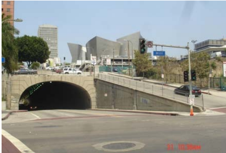
Figure 4-13. East End of 2 nd Street Tunnel
