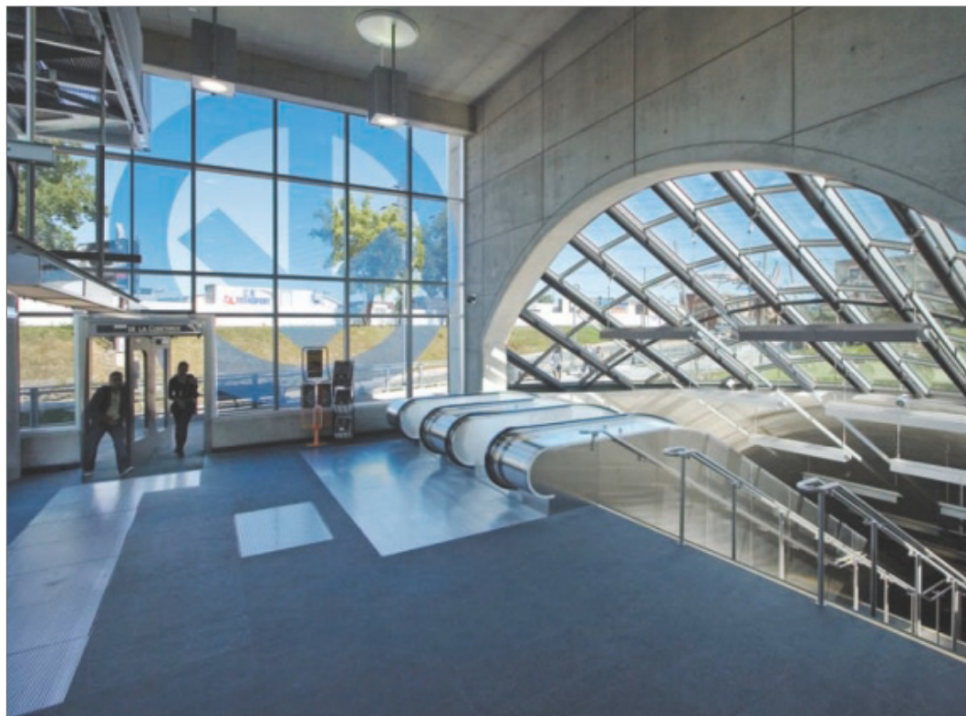
◀ Train Portal Structure
