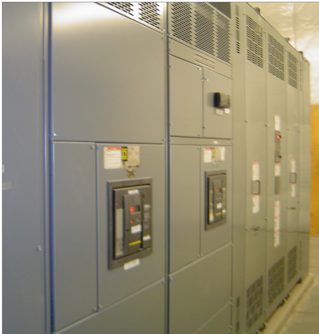
◀ Secured ancillary facilities must be provided accordingly.
