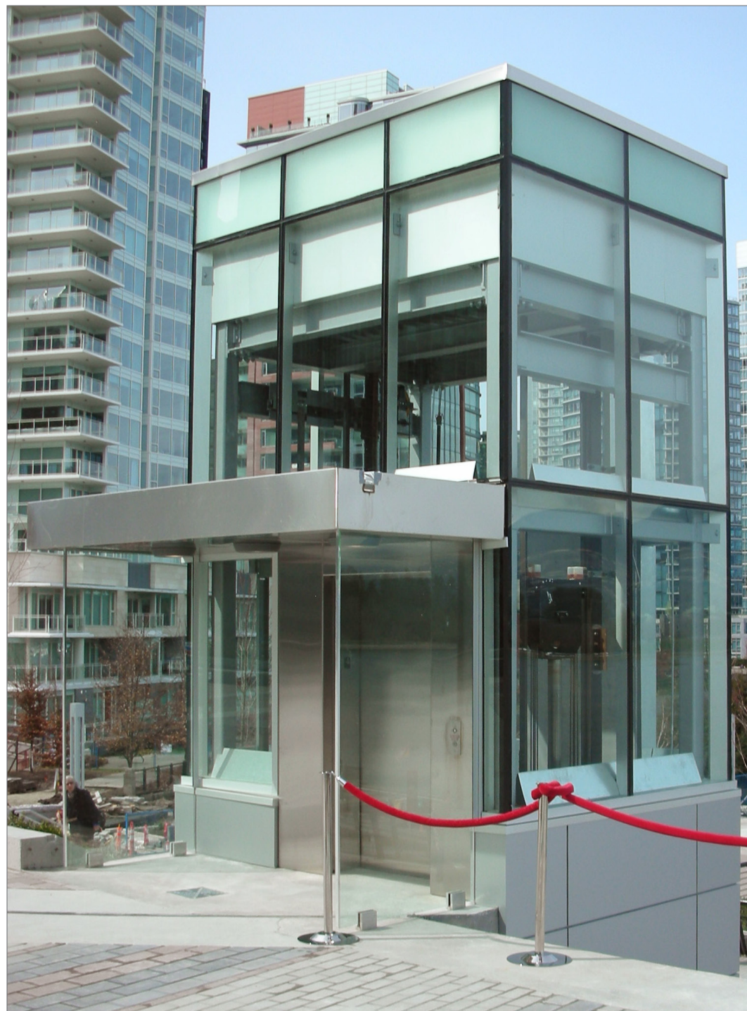
◀ Elevators increase accessibility to underground stations.
