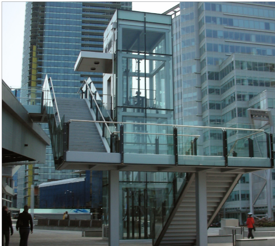
◀ Safe and efficient vertical station circulation.
