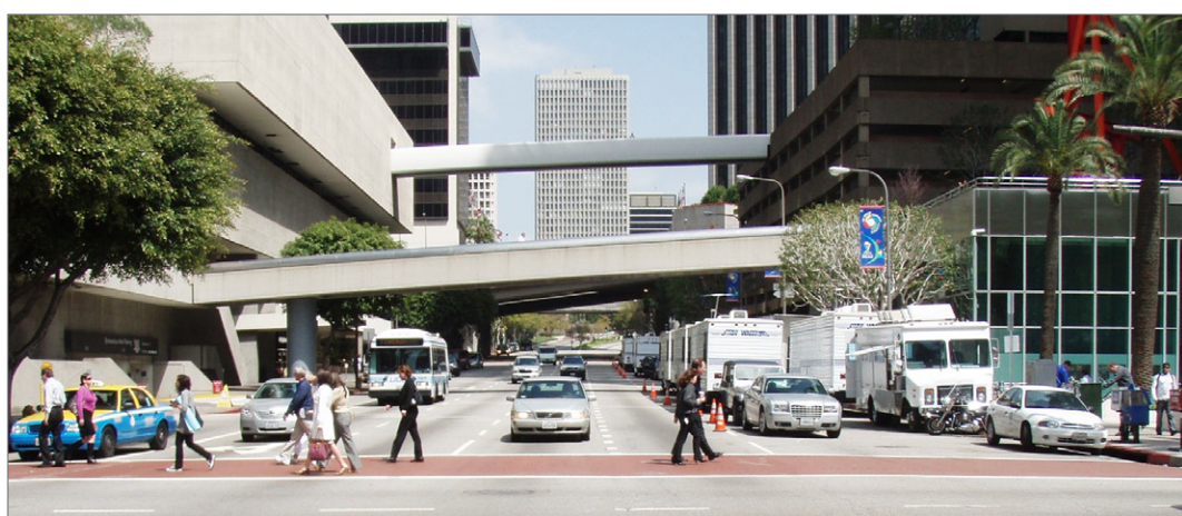
◀ Financial District – Existing Streetscape
