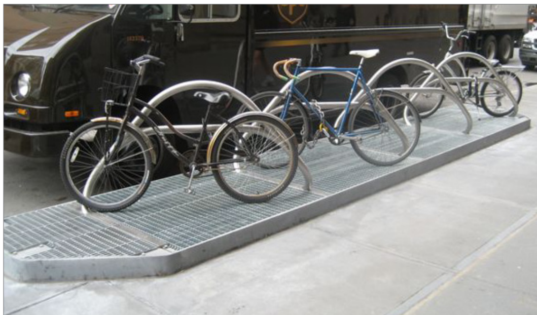
◀ Bike racks present an opportunity to reflect the character of the local community through their design. This bicycle rack is integrated with the metal grate / ventilation shaft.
