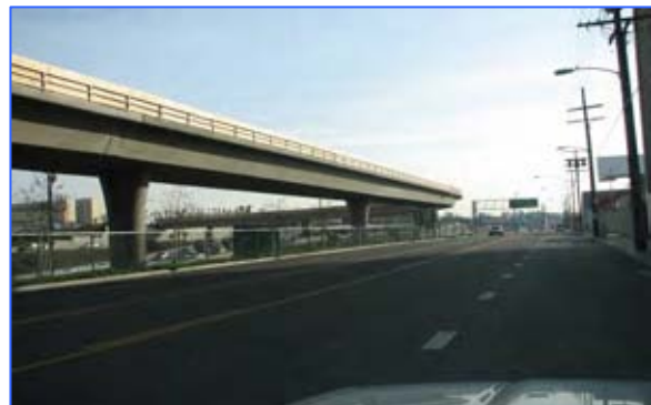
Figure 2-4 LRT Bridge over US-101
