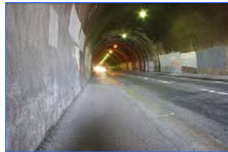
Figure 2-6 3 rd St. Tunnel
