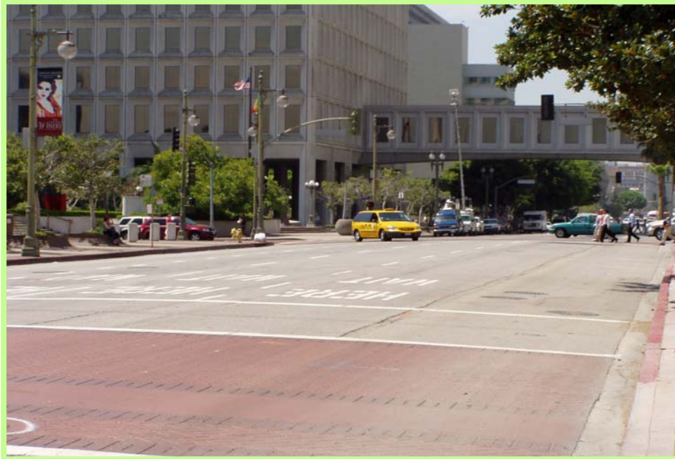
Main St. at Temple, Looking South – Before
