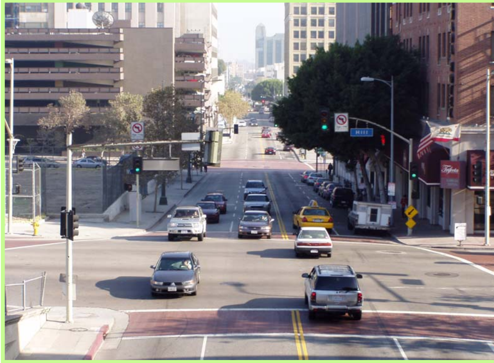
2 nd and Hill, Looking East - Before
