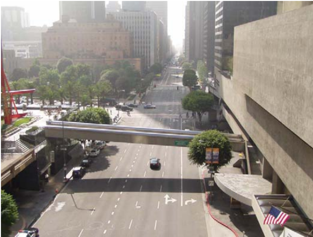
Wide roadway on Flower Street near 5 th Street, with six automobile traffic lanes and one curb lane of parking. This segment of Flower Street carries about 20,000 cars on a typical weekday.
