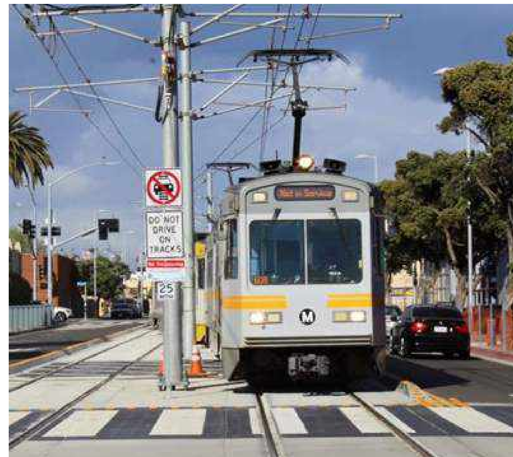
At-Grade: Expo Line – Santa Monica
