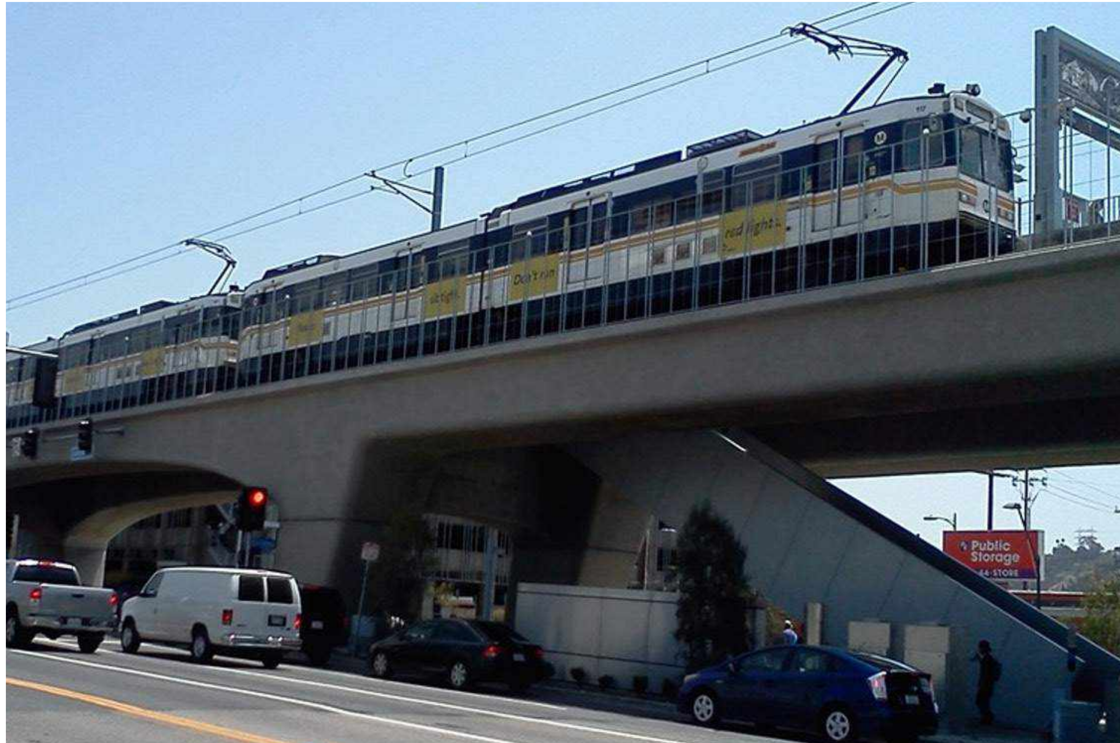
Elevated: Expo Line – La Cienega
