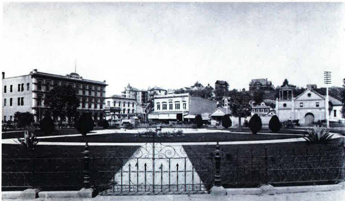
Figure 4. The Plaza as it appeared in 1890. (Source: Los Angeles Public Library).
