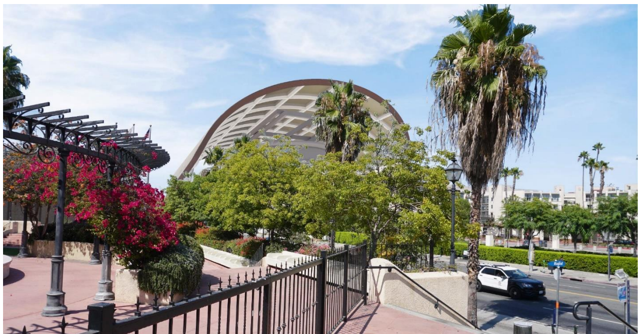
Figure 45: View of Alameda Station looking east from Placita de Dolores. RIOS, 2021.
