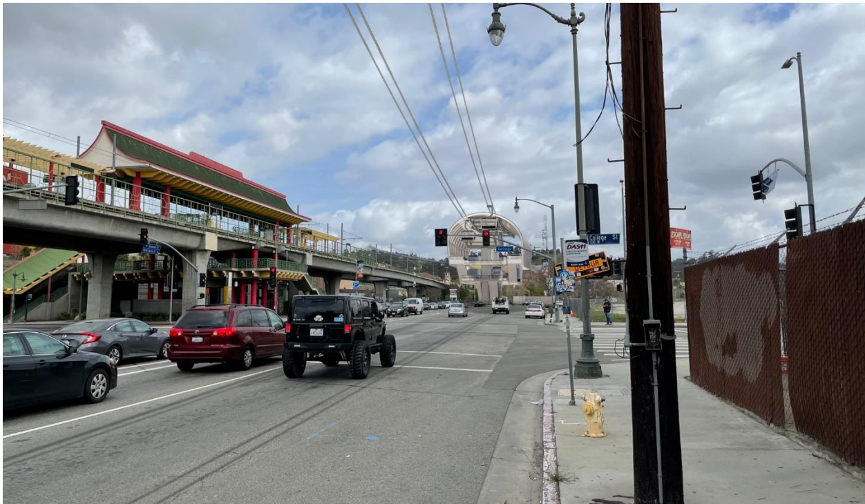
Figure 49: View of Chinatown/State Park Station, looking north on Spring Street adjacent to Metro L Line (Gold) Chinatown Station. RIOS, 2022.
