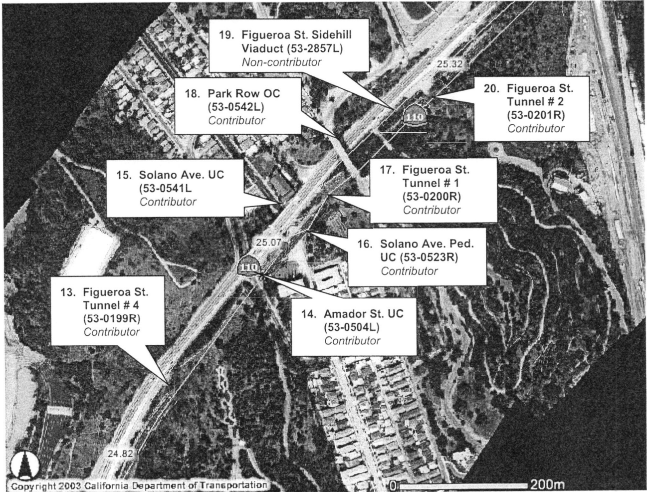
Arroyo Seco Parkway Historic District Segment C
