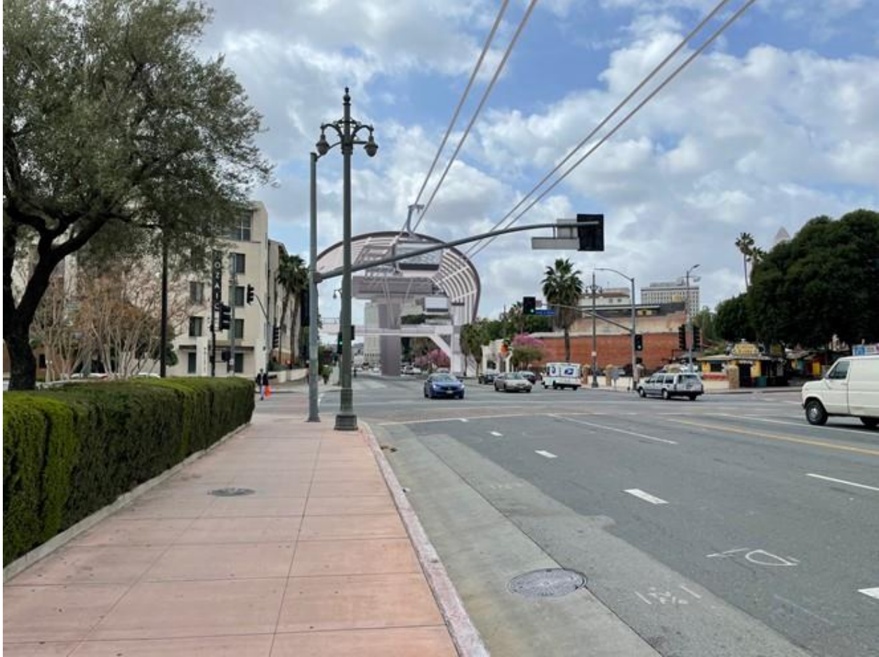
Figure 43: View of Alameda Station looking south on Alameda Street from just north of Cesar E. Chavez Avenue. RIOS, 2021.
