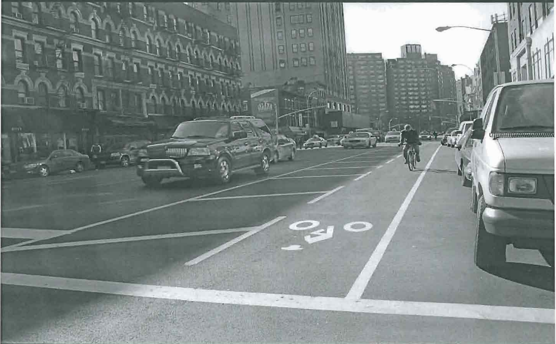
8 th Avenue, Manhattan – Buffered bicycle lane, 3 vehicle lanes
