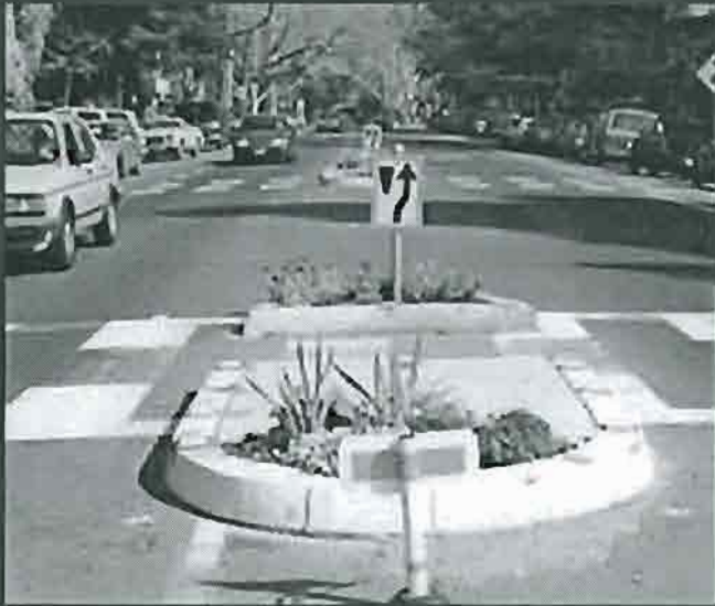
Pedestrian island with 'cut-through'
